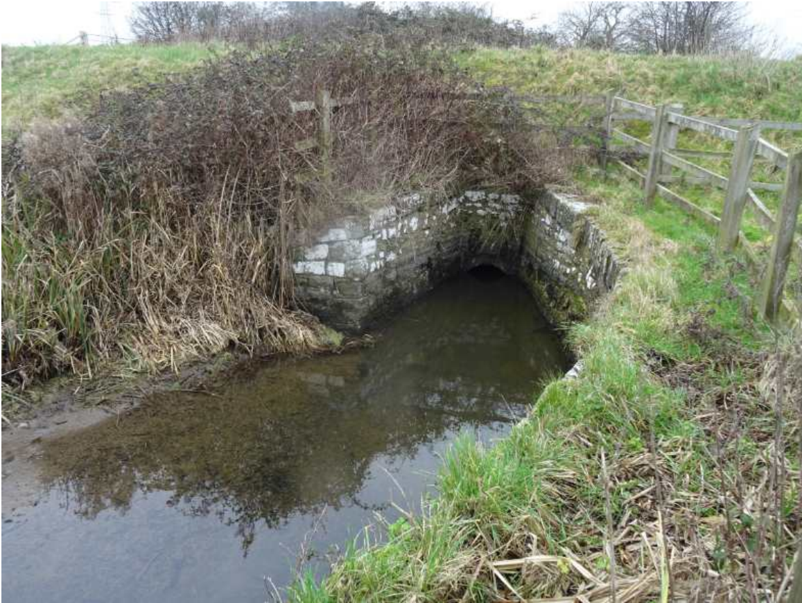
Fig 17: Rennie's siphon, southern (exit) end. Note anti-erosion extended curving cheek wall
