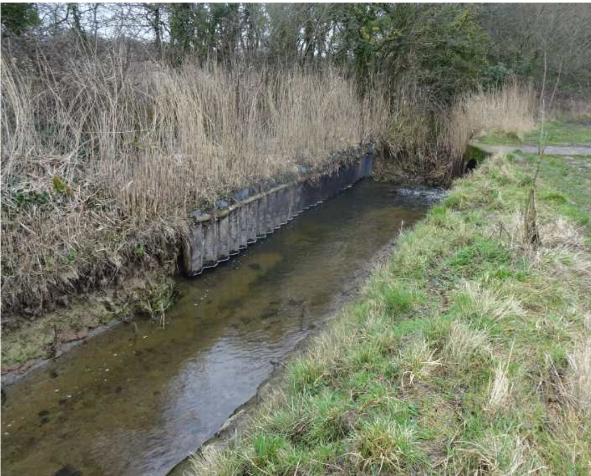
Fig 14: Anti-erosion measures at the junction of the New Rhyne and Binhay Rhyne
