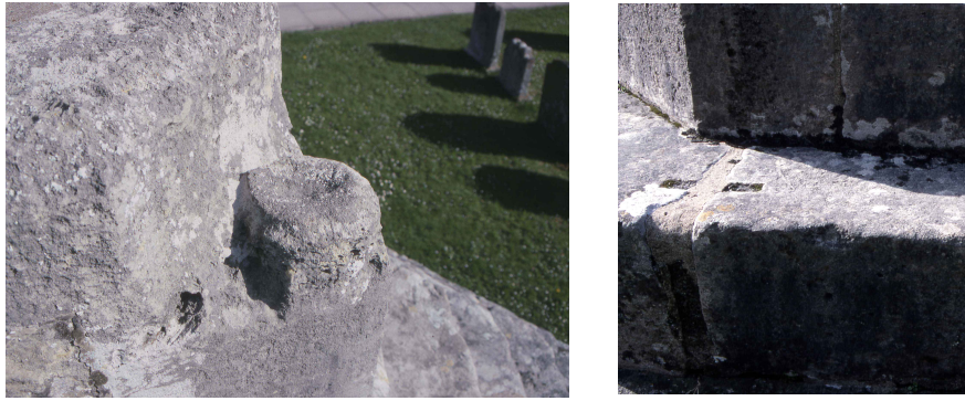
Fig 6: Dowelled feature on socket and cramp socket on step
