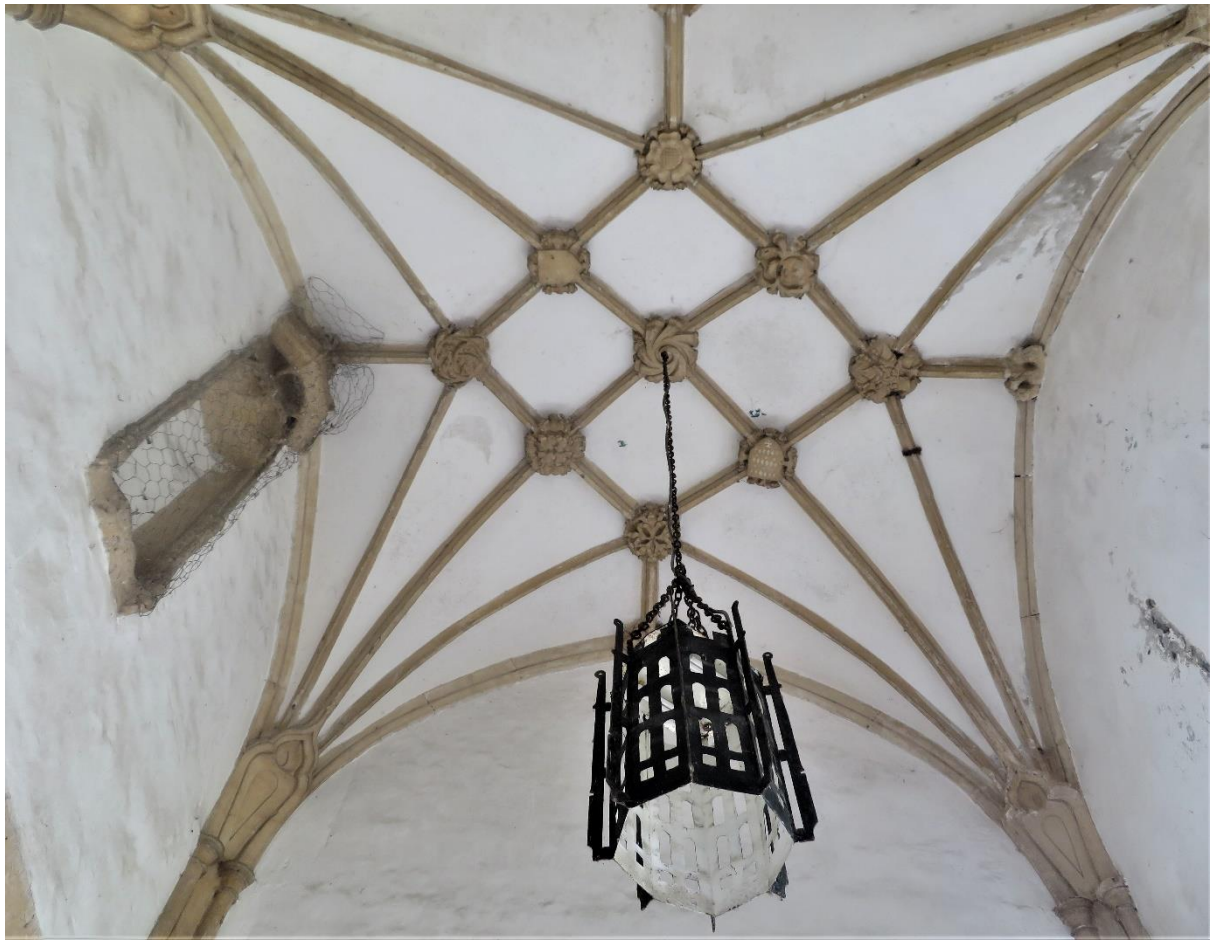
The ceiling is a thin-ribbed lierne-vault containing nine moulded bosses. The bosses contain foliage, shields and a green man.
