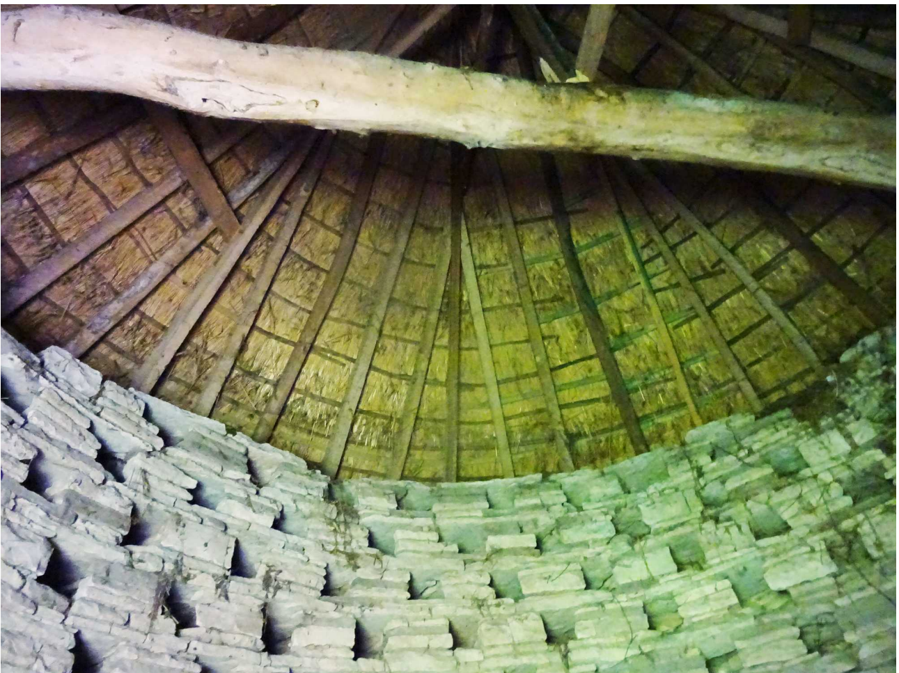
Interior of medieval dovecote, Ham Farm
