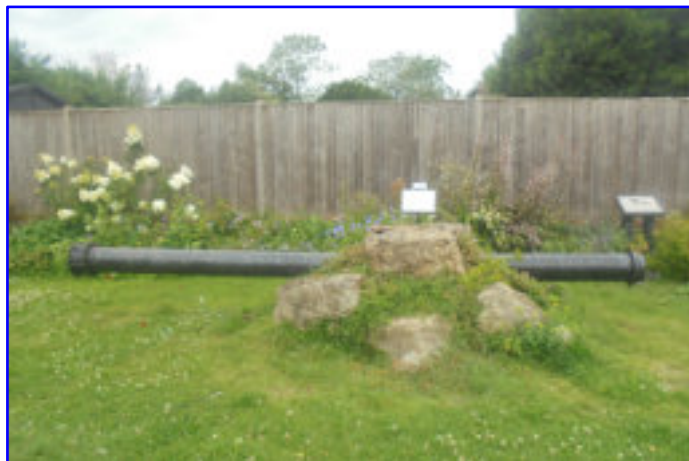
Section of the PLUTO pipeline at Marden
