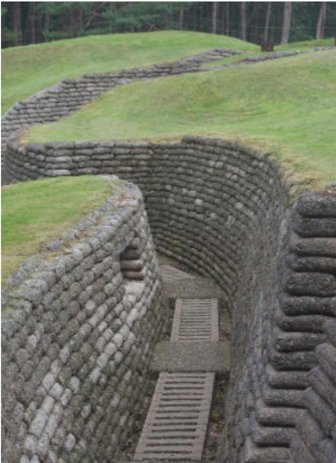
The shell holes are clearly visible in the grass. In one area, the trench outlines have been made more permanent by the addition of concrete “sandbags”.
