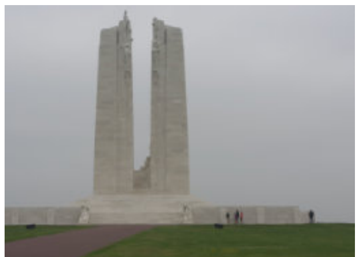
The two pylons which tower above the ridge line and the 20 sculpted allegorical figures are made from almost 6,000 tonnes of limestone.
