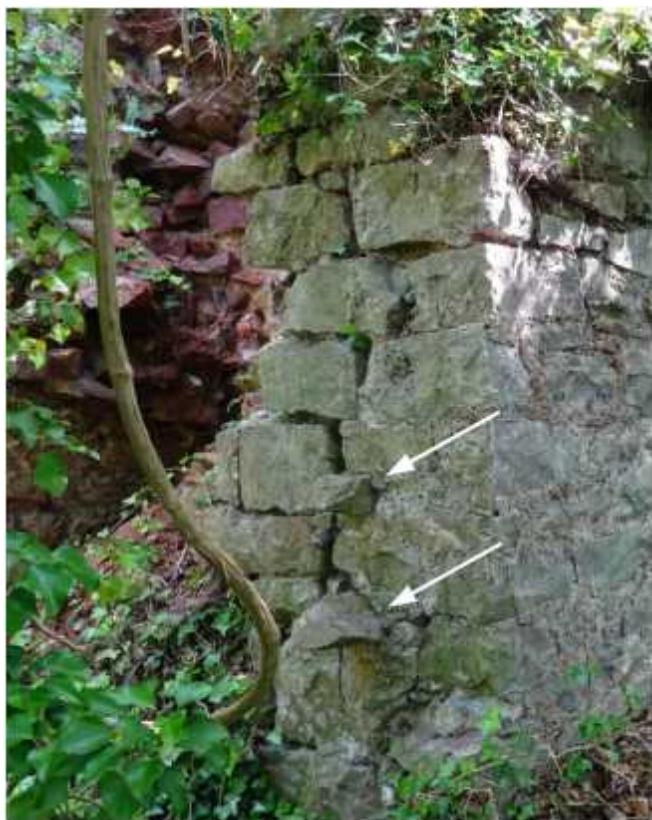
Fig 6: South side of West kiln, showing key stones for cheek wall projecting from the body of the kiln (arrowed)
