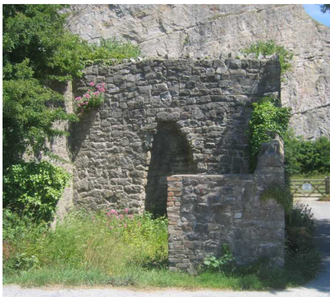
Fig 5: Limekiln at Uphill quarry (ST31515839) showing cheek walls surviving in front of the kiln face
