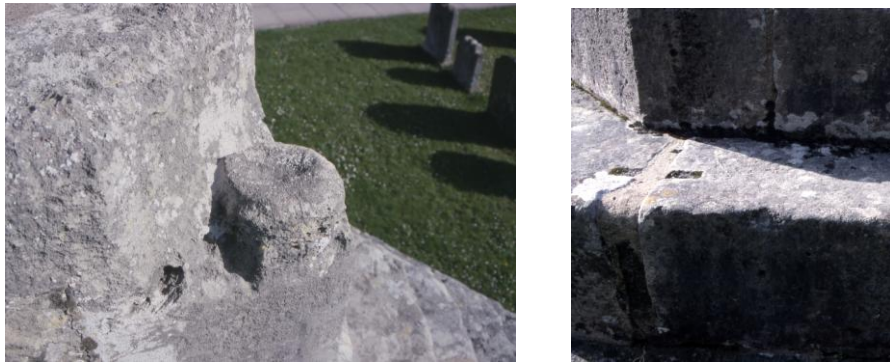
Fig 5: Dowelled feature on socket and cramp socket on step
