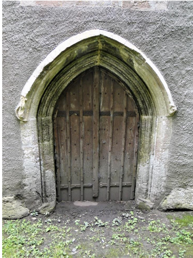
The west door to the tower has a moulded two-centred arched head with a dripstone over it.
