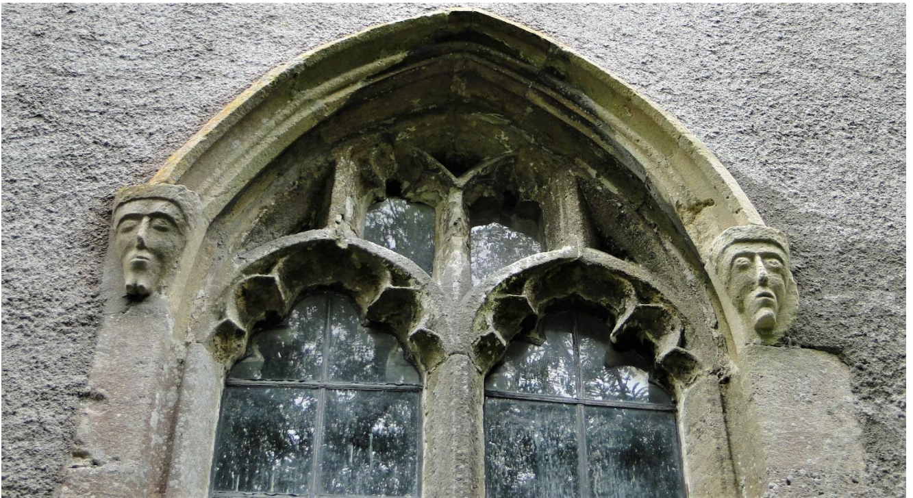
This has cinquefoil heads to each light and reticulated tracery and also a heavy dripstone with head terminals.
