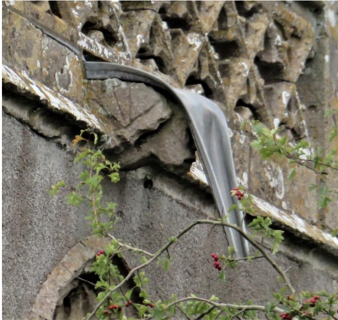
The west side has a central gargoyle draining the roof.
