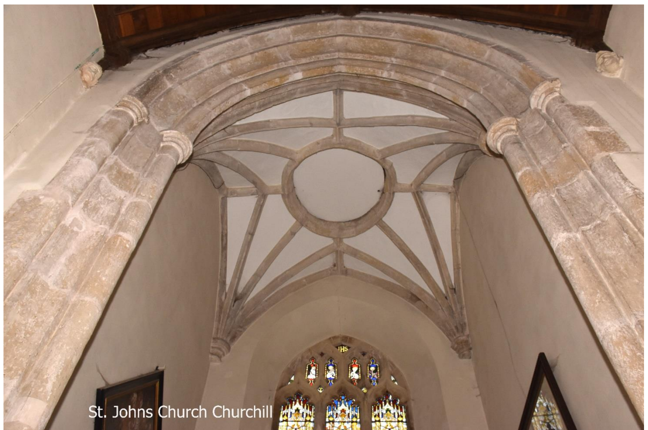
Fig 14: The fan vault and bell access hatch, tower ceiling.
