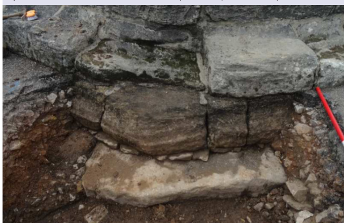
The basement and lowest step of the cross with chock stones between, 03 August (sorry it's a bit grubby and needs tidying, but we'll be doing that tomorrow).
