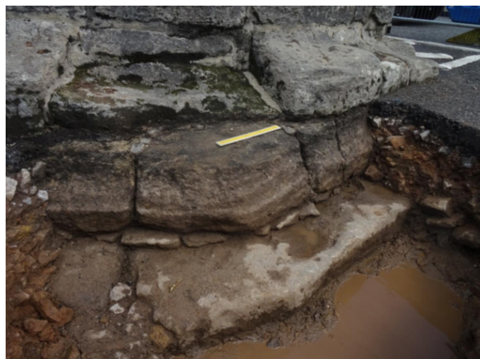
Excavation showing one of the large basement stones with first step stones chocked level with small stones.
