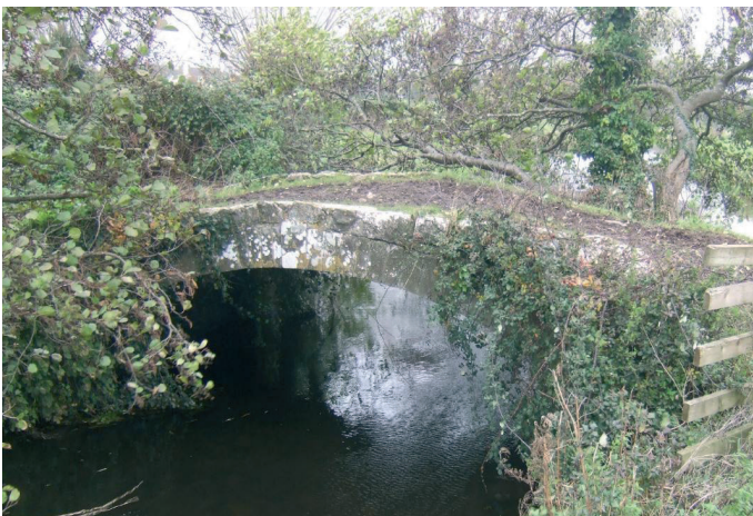
Fig 4: The Listed bow (bridge) at the Park, Congresbury: note the one stone deep parapet, which the others don't have
