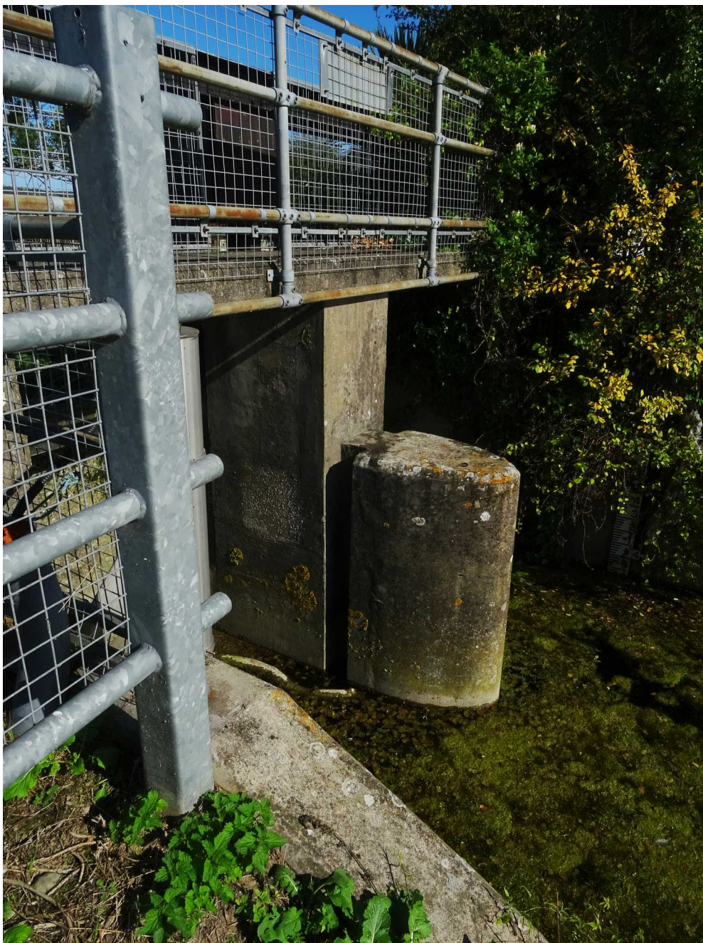
Fig 6: Kenn Pier Sluice, diverting potential flood water from the Kenn River at the west end of Nailsea Wall, into the Blind Yeo, constructed mid-20th century
