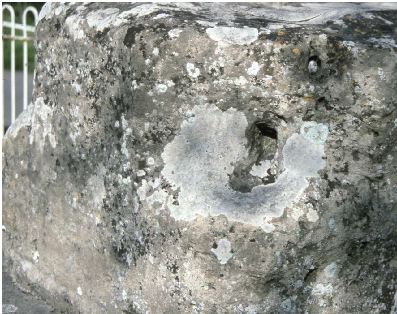
Fig 10: The square socket replacing the missing stop-chamfered
