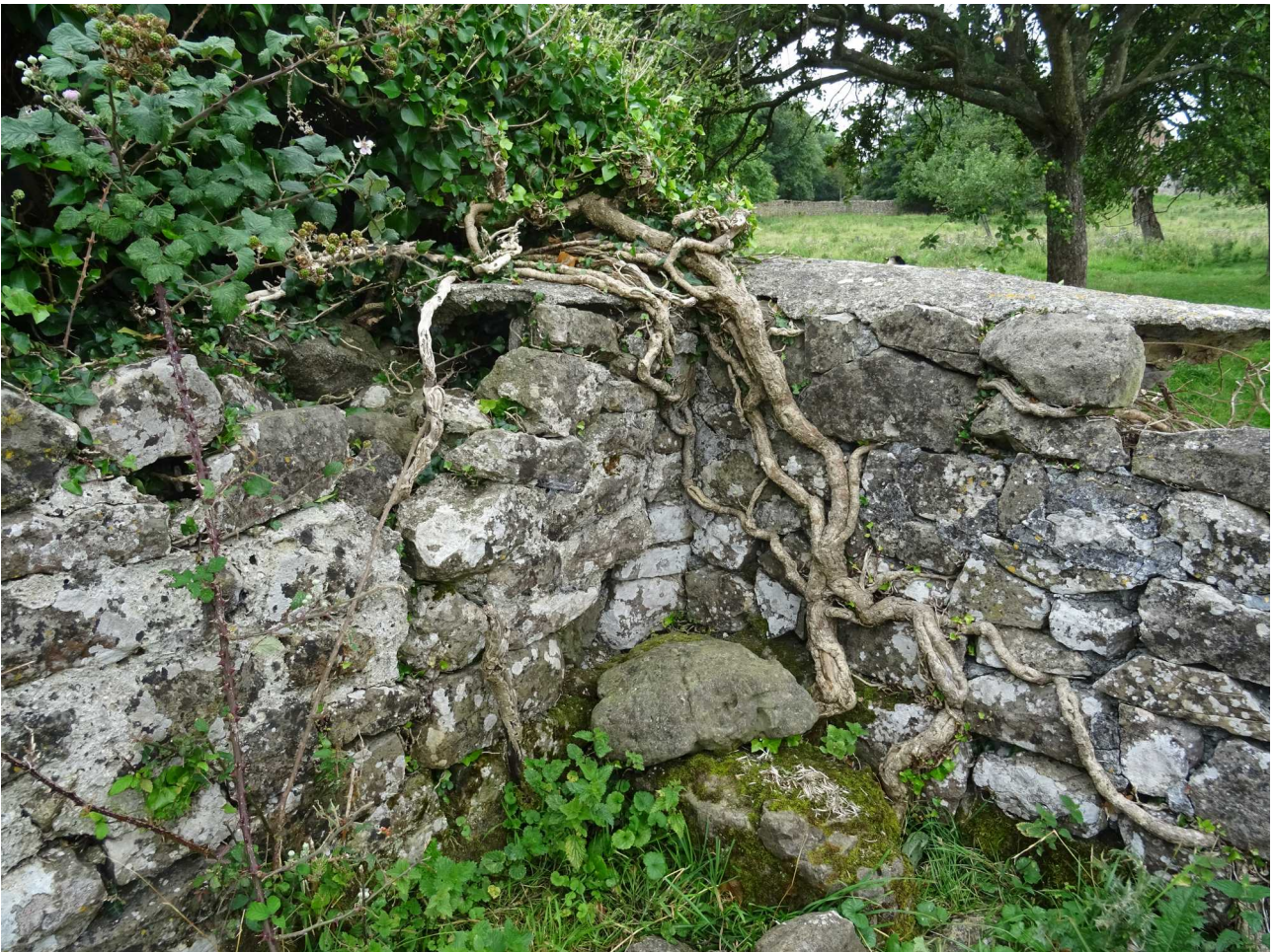
Junction of orchard wall with earlier, close to site
