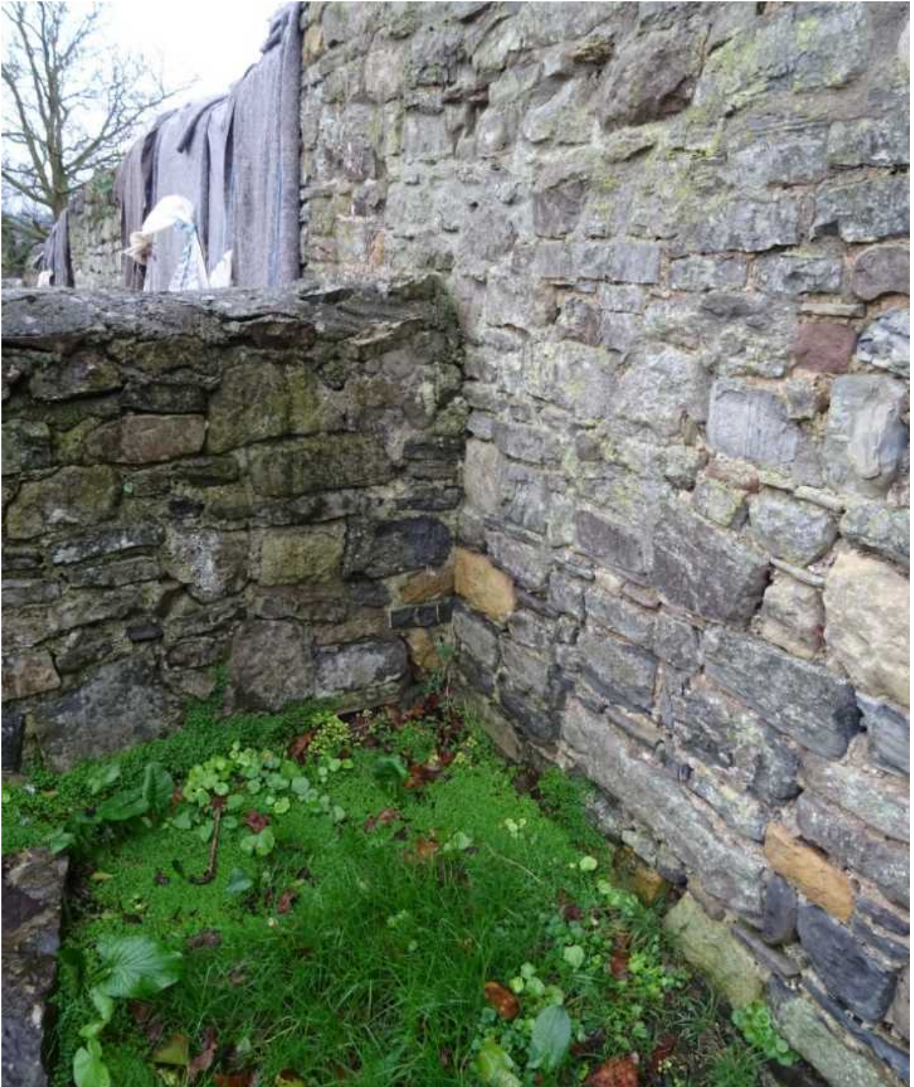
Fig 80: Wall 12/15 junction with wall 11, indicating more regular basal courses and potentially less regular courses above (the same can be seen on the cover illustration)
