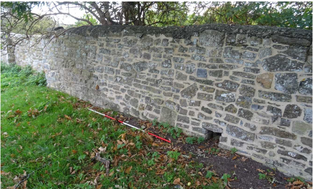
Fig 114: Wall 18, north side, east end, completely repaired and repointed
