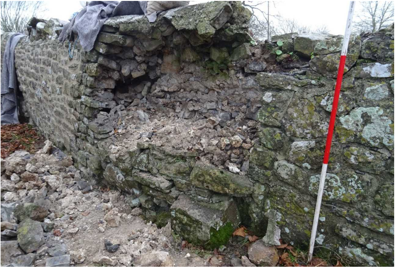
Fig 124: Central portion of wall 19 (from east): this was unstable, and had to be rebuilt
