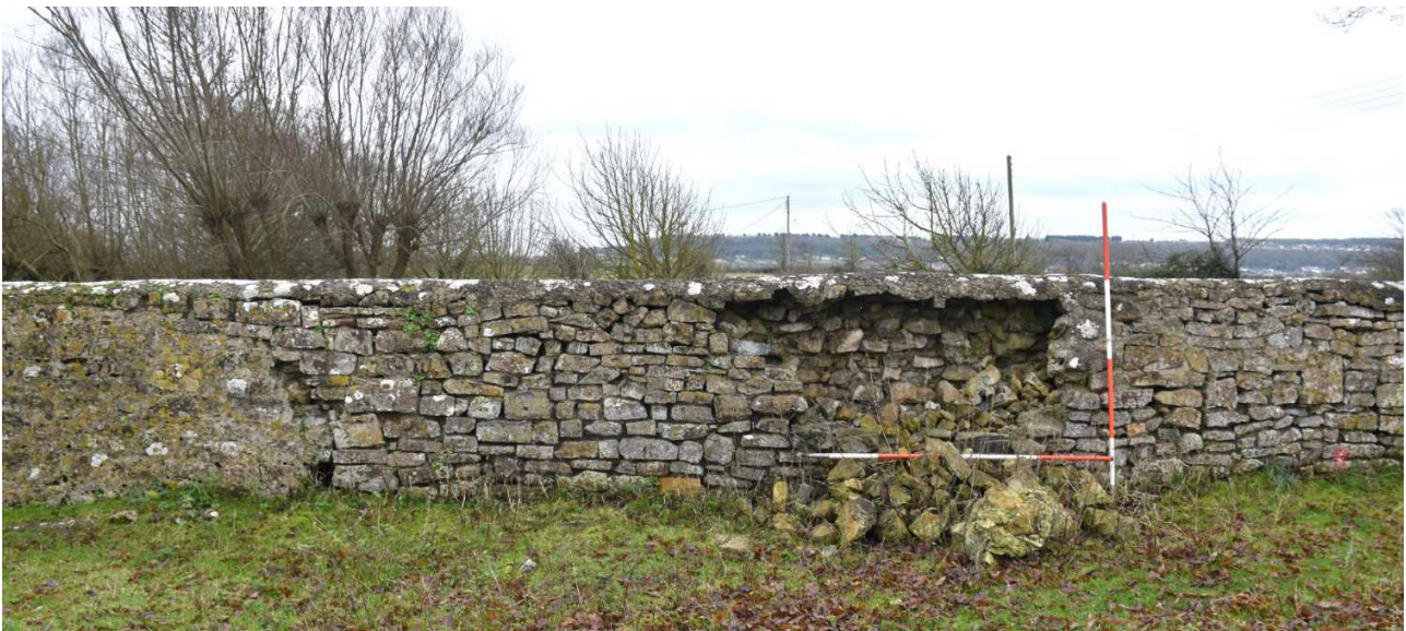
Fig 106: Larger collapse (ii) under concrete wall topping, towards the centre of the wall (2020)
