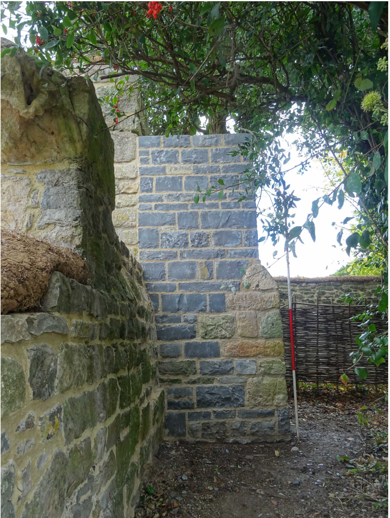
Fig 87: New buttress (2022) and repointed south side of wall/structure 13
