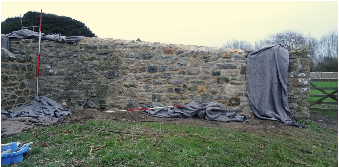
Fig 97: Repaired wall collapse and repointing, wall 17 north of field gate, 2022
