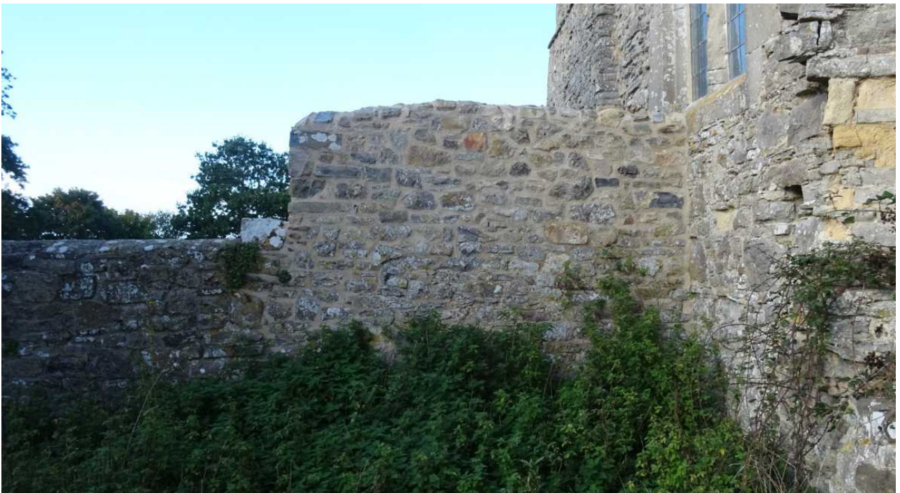
Fig 125: Rebuilt and repointed north end of wall 19
