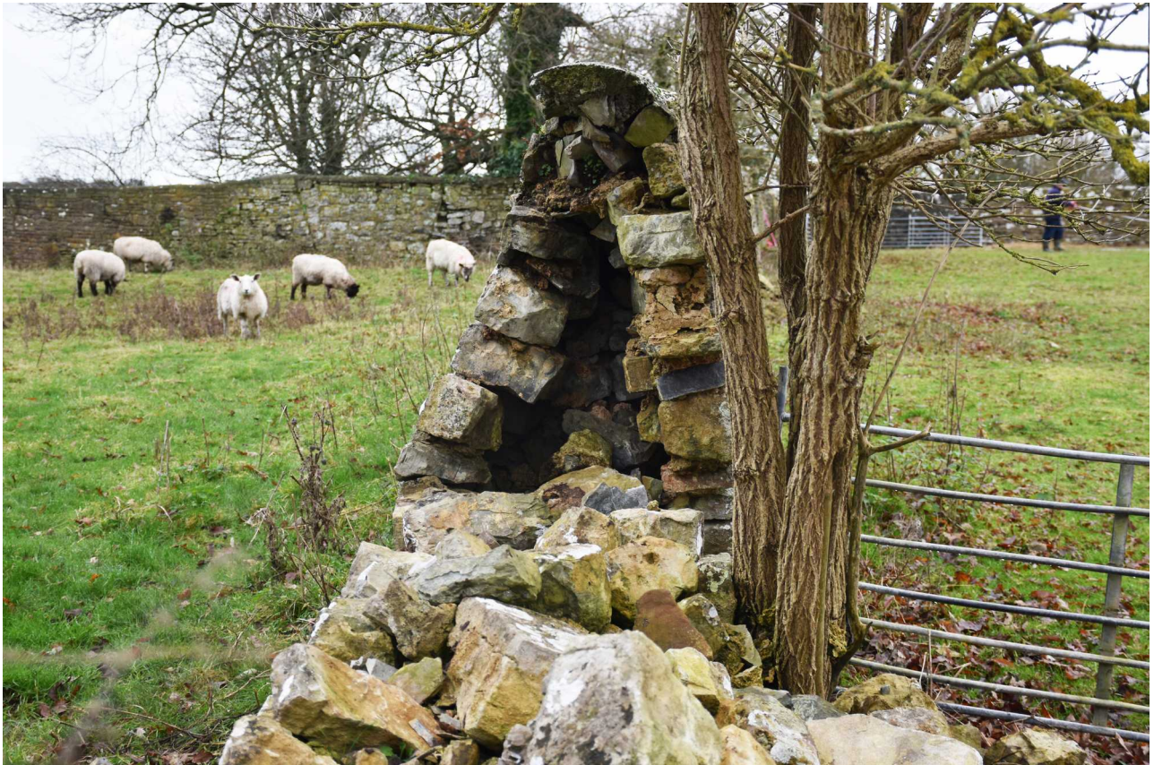
Fig 102: 'Double-skinned' structure of wall 18, seen in collapse at its eastern end, 2020
