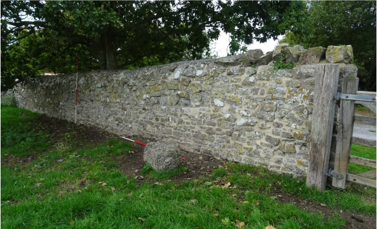
Fig 98: Wall 17 south of gate repointed 2022
