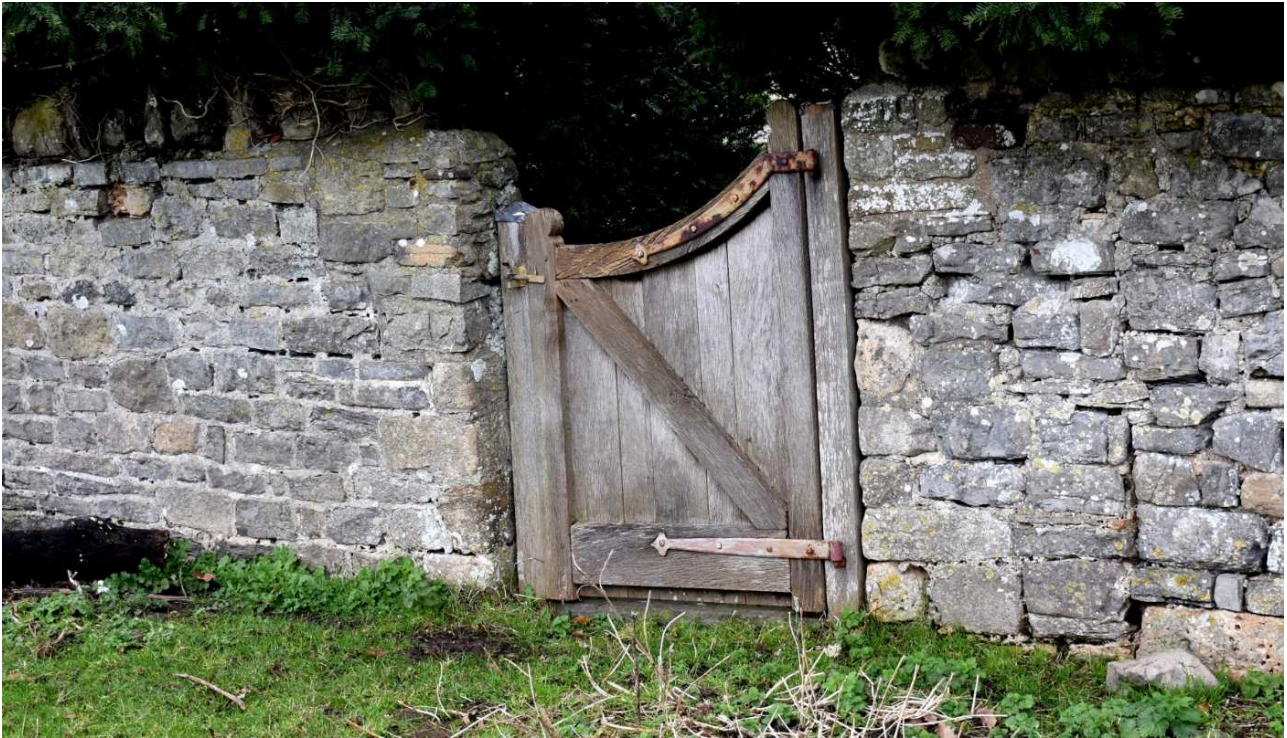
Fig 74: Current gate in wall 11, with clear evidence of filling in of a former wider gateway to its east
