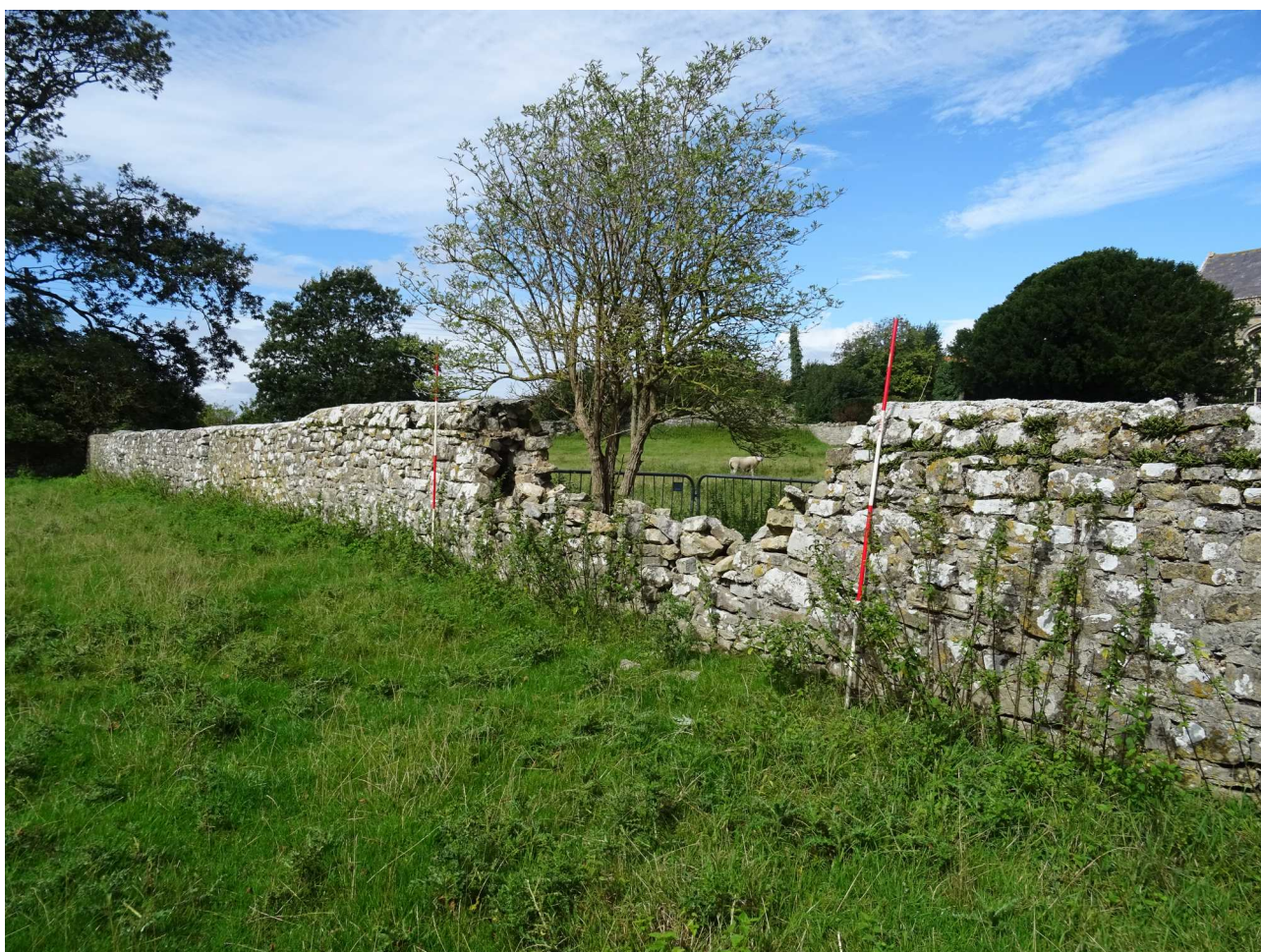
Fig 101: Wall 18 (2020) showing patched nature of wall and major collapse
