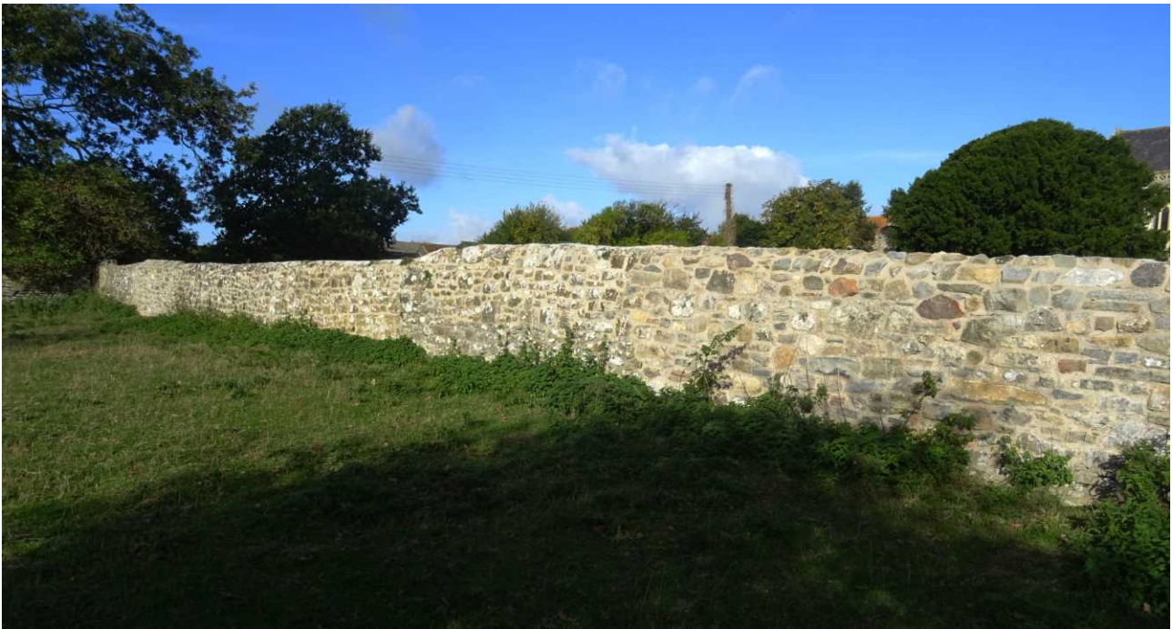
Fig 113: Wall 18, south side, completely repaired and repointed (2022)
