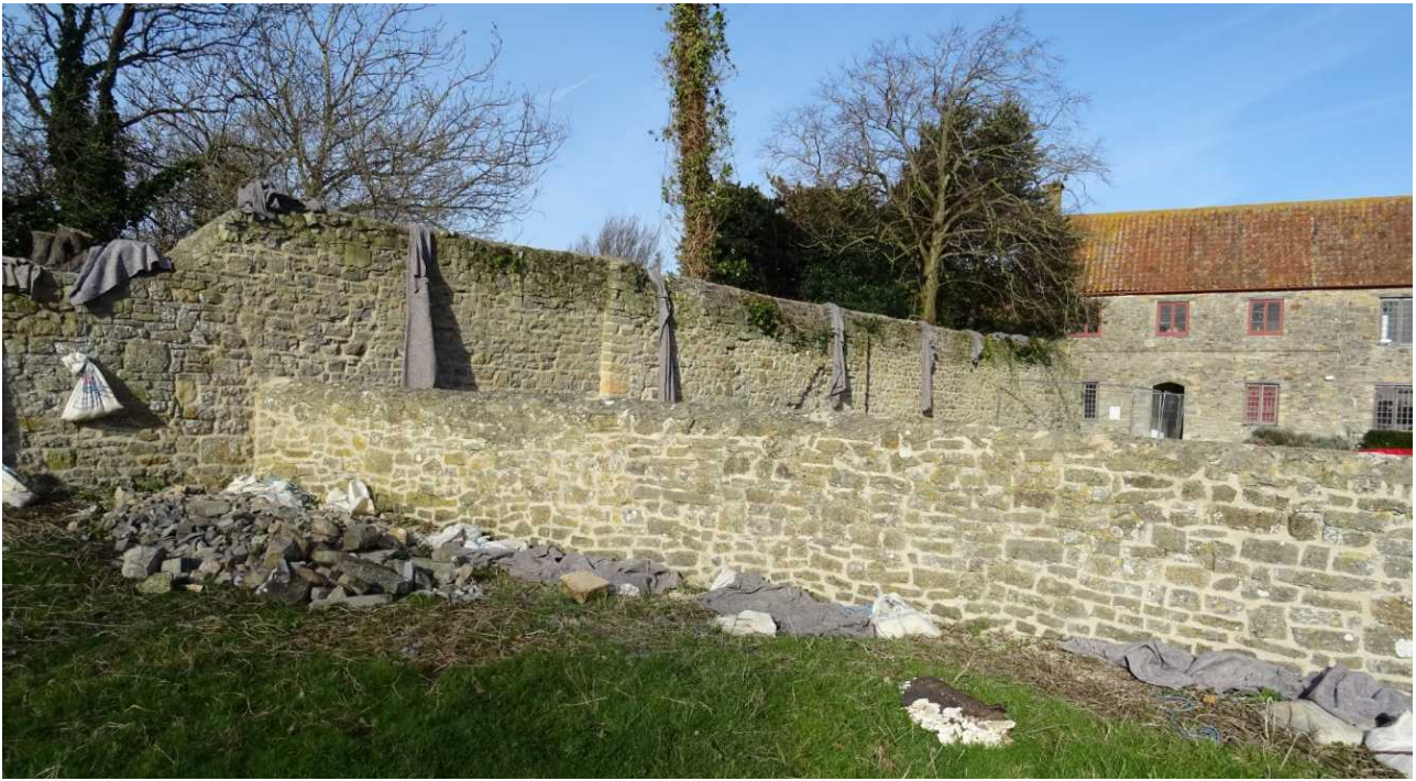
Fig 76: Wall 11 successfully repointed, 2022
