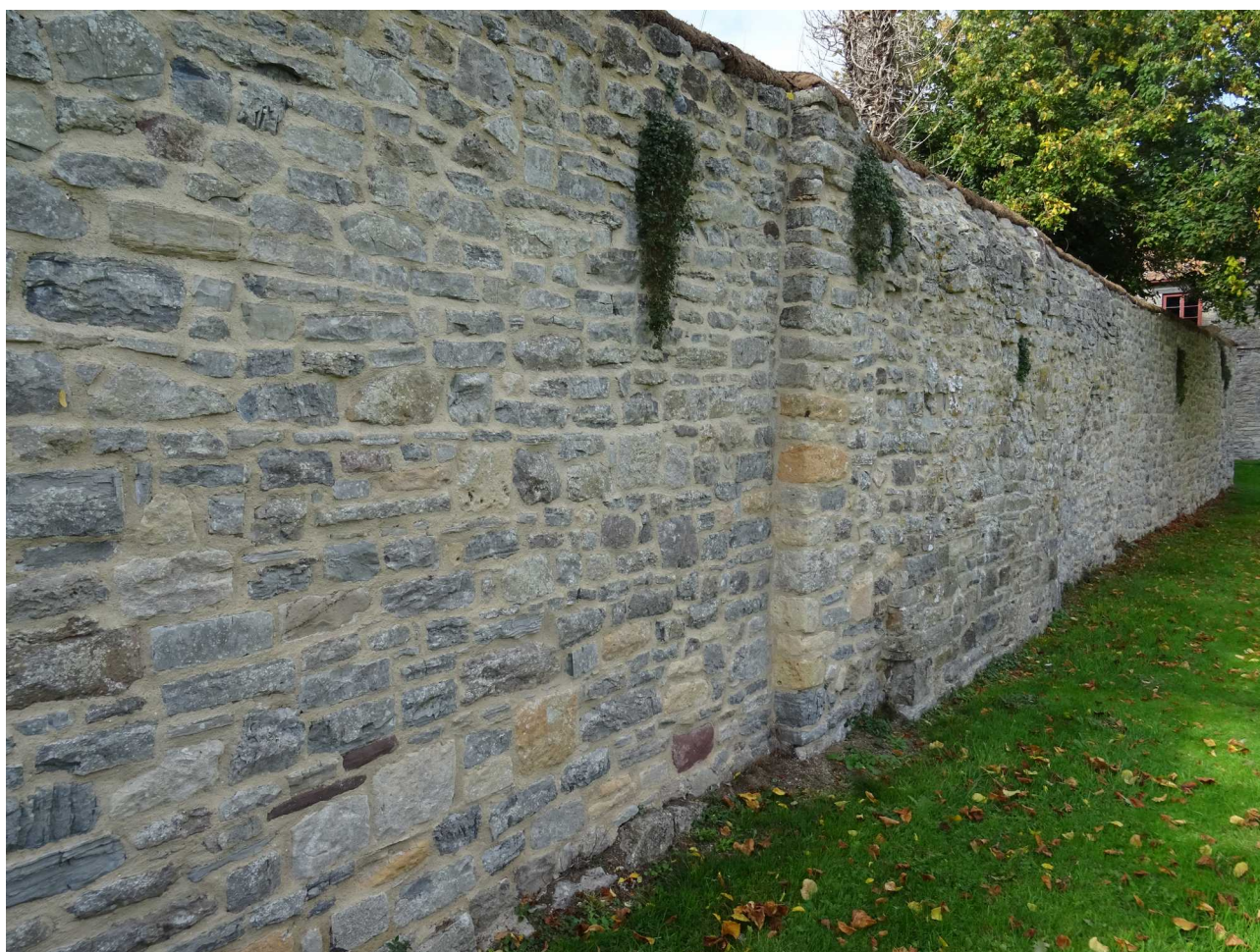
Fig 79: Thickening of wall 12/15 on its eastern side (after repairs, 2022)
