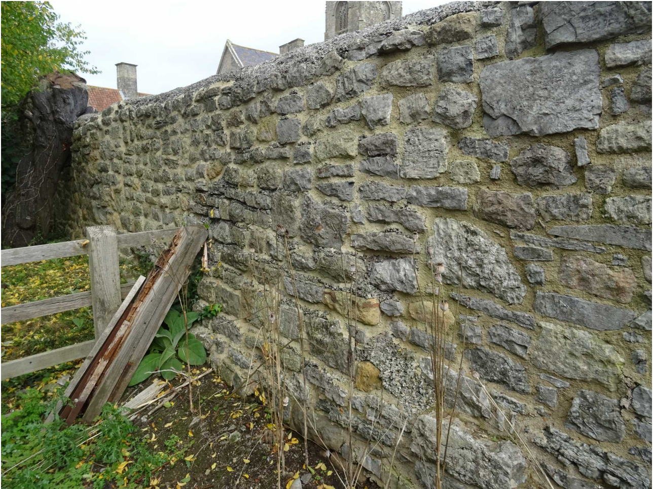
Fig 81: Repointing at southern end of wall 15 (2022)
