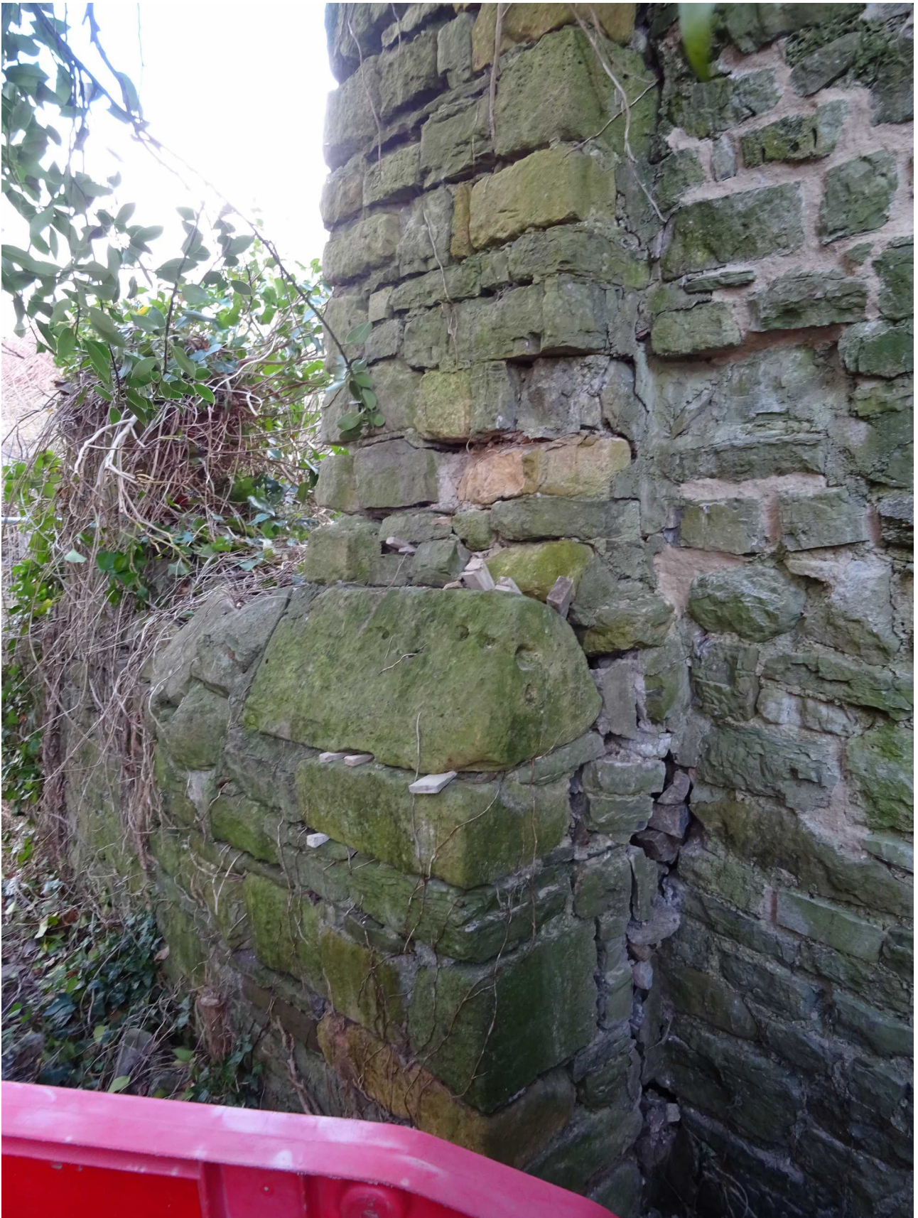
Fig 86: Butt joint of walls 13 and 14 (Feb 2022), showing failure and movement of the south part of 13.
