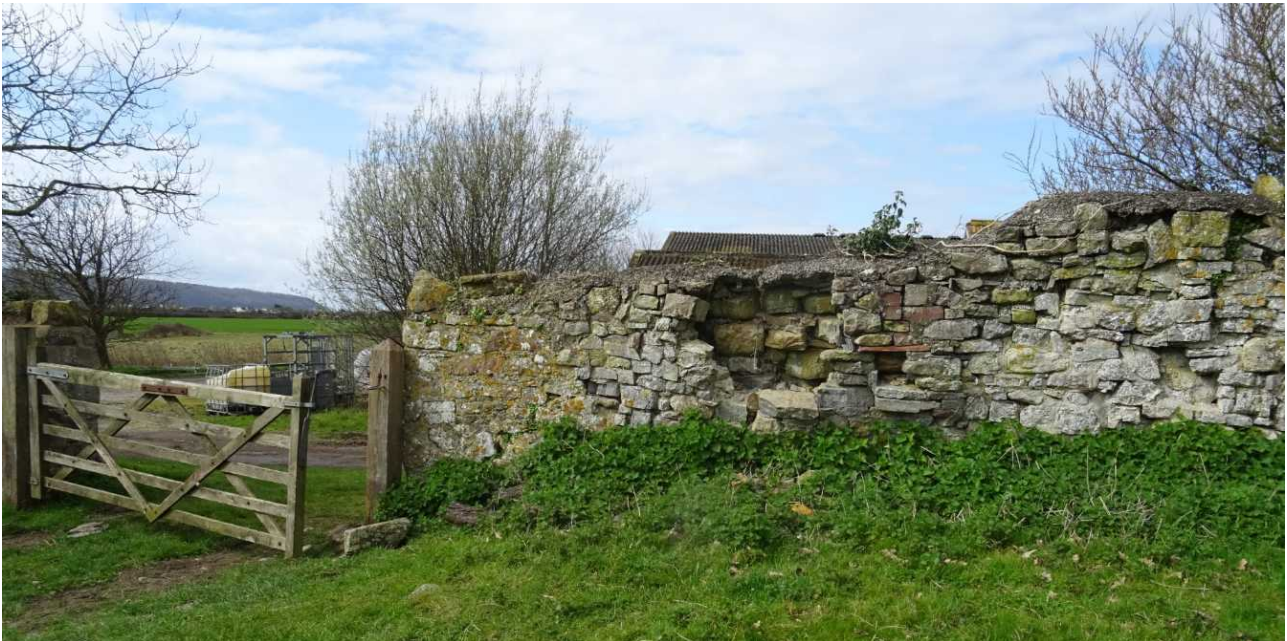
Fig 94: Wall gate and collapse in wall 17 (2021)
