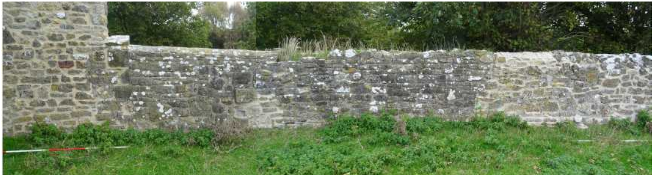
Fig 126: Exterior (east) of wall 19 after rebuild and repointing (2022)
