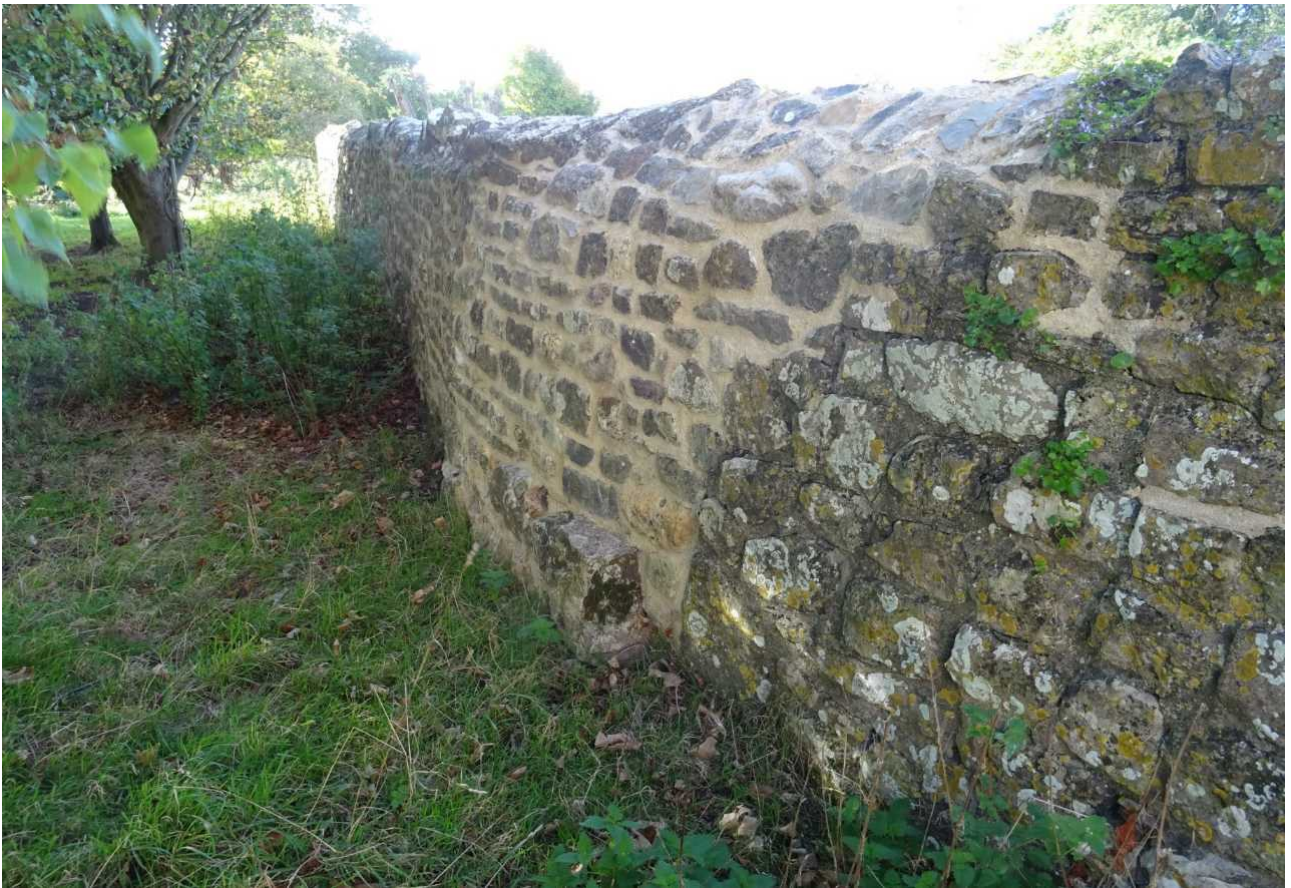
Fig 126: Exterior (east) of wall 19 after rebuild and repointing (2022)
