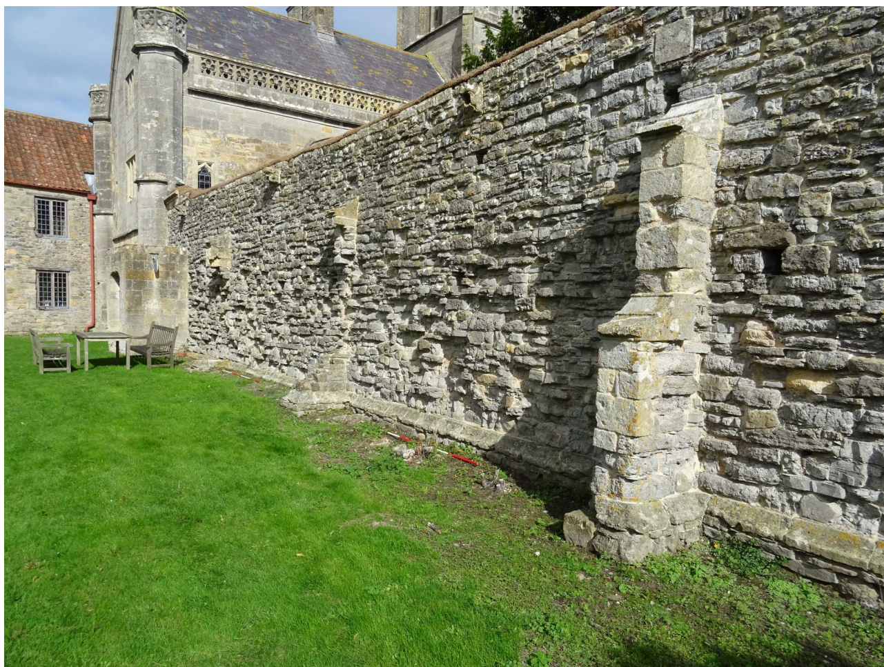
Fig 60: Northern (external) view of wall 10, after repairs, 2022 - note buttresses, gargoyles and basal string course
