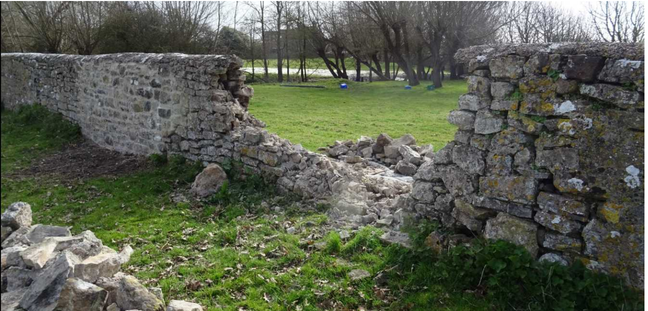
Fig 108: Collapse ii, cleared for rebuilding (2020) other area of major repair alongside to left)
