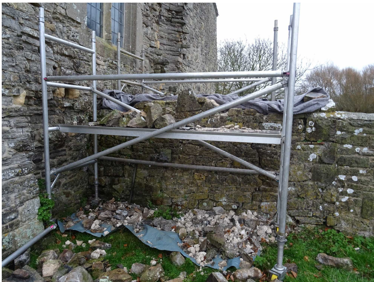
Fig 123: Works underway to rebuild part of wall 19 against the infirmary (late 2021)
