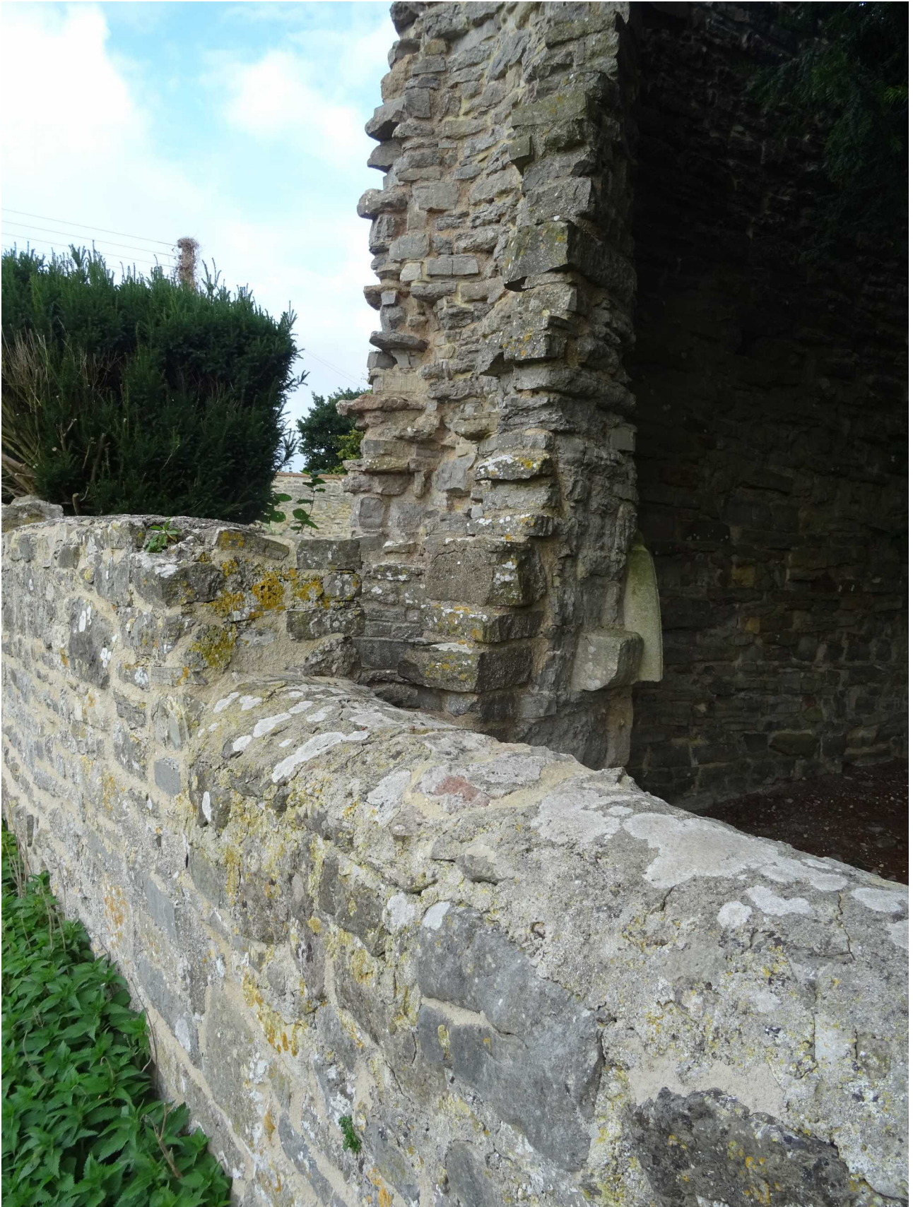
Fig 69: Junction of walls 9, 10 and 11 after repointing works, 2022
