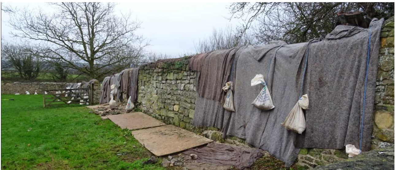
Fig 93: Wall 17 under repair and frost protection (2022)
