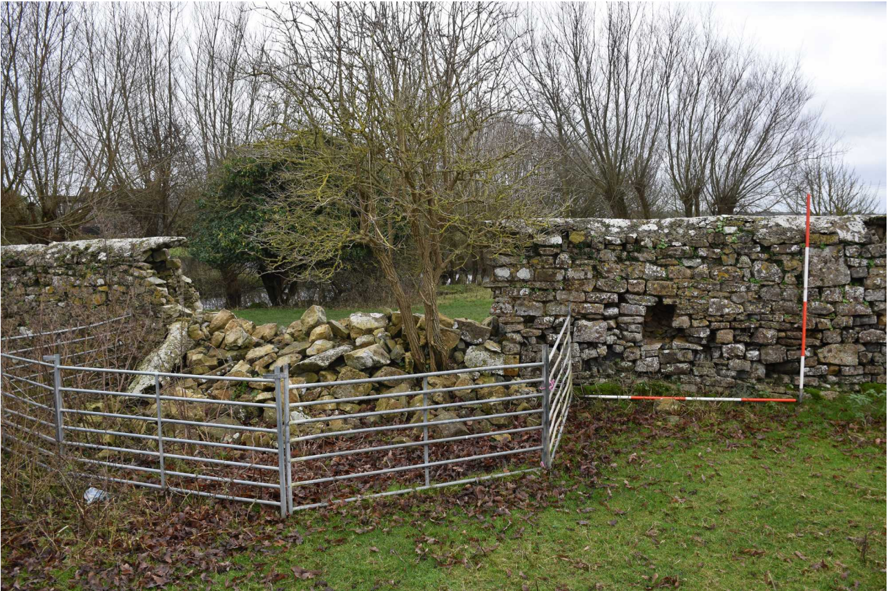
Fig 107: Large collapse (iii) close to junction of wall 18 with wall 19 (2020)
