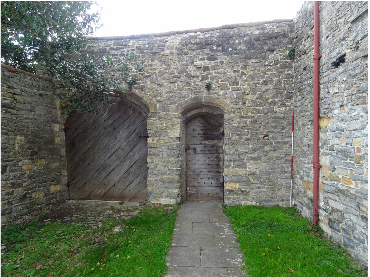
Fig 88: East (inside) of wall 13 after repointing, 2022 (note the absence of freestone jambs to either opening)
