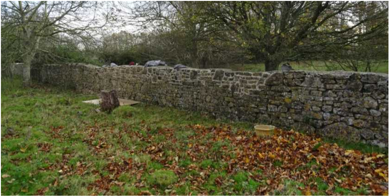
Fig 31: Section of wall as seen in Fig 30 (above) after repointing
