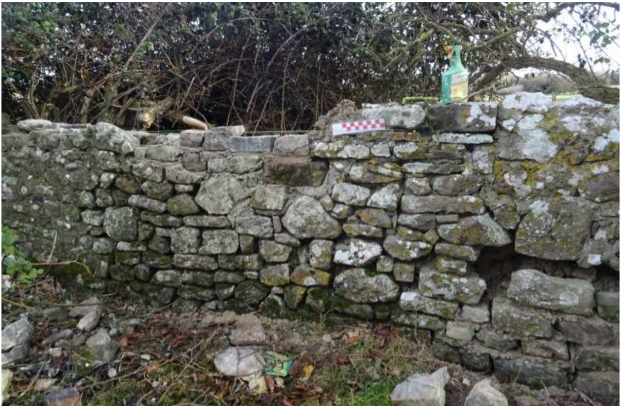
Fig 27: Formerly overgrown collapse of wall 4 close to junction with wall 3 under repair
