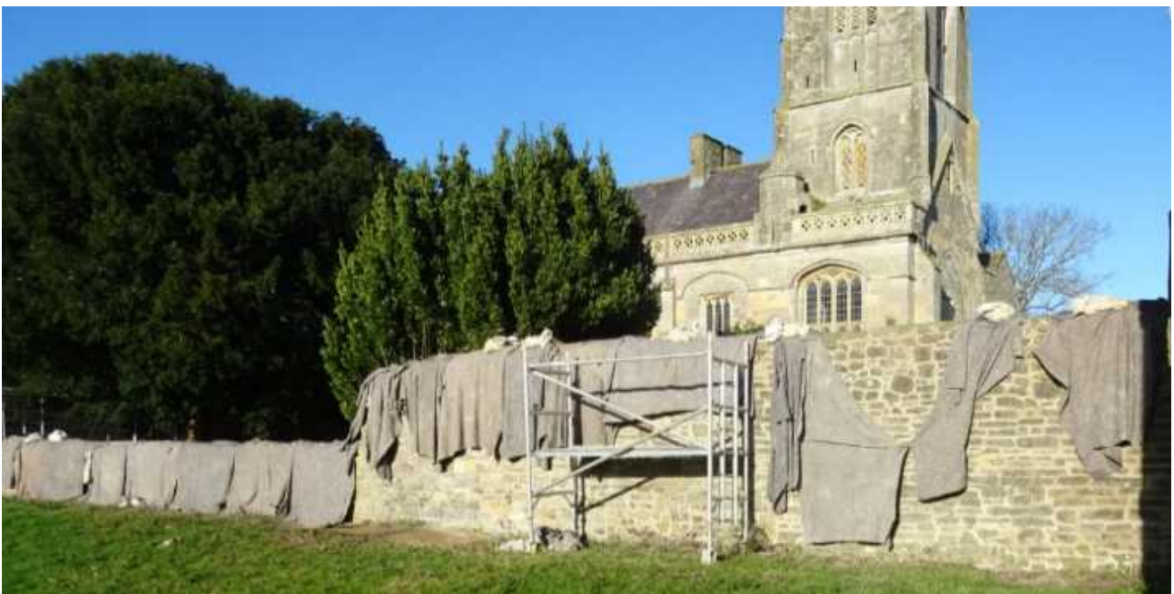
Fig 39: Wall 6 during repointing works, 2022
