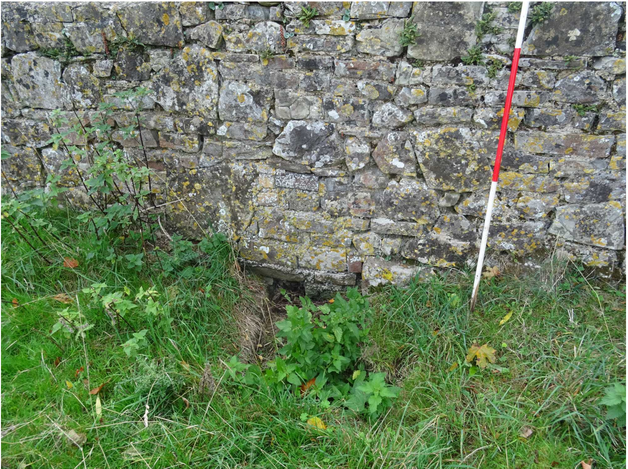
Fig 34: Drain hole from orchard under wall 5 (one of at least three present)
