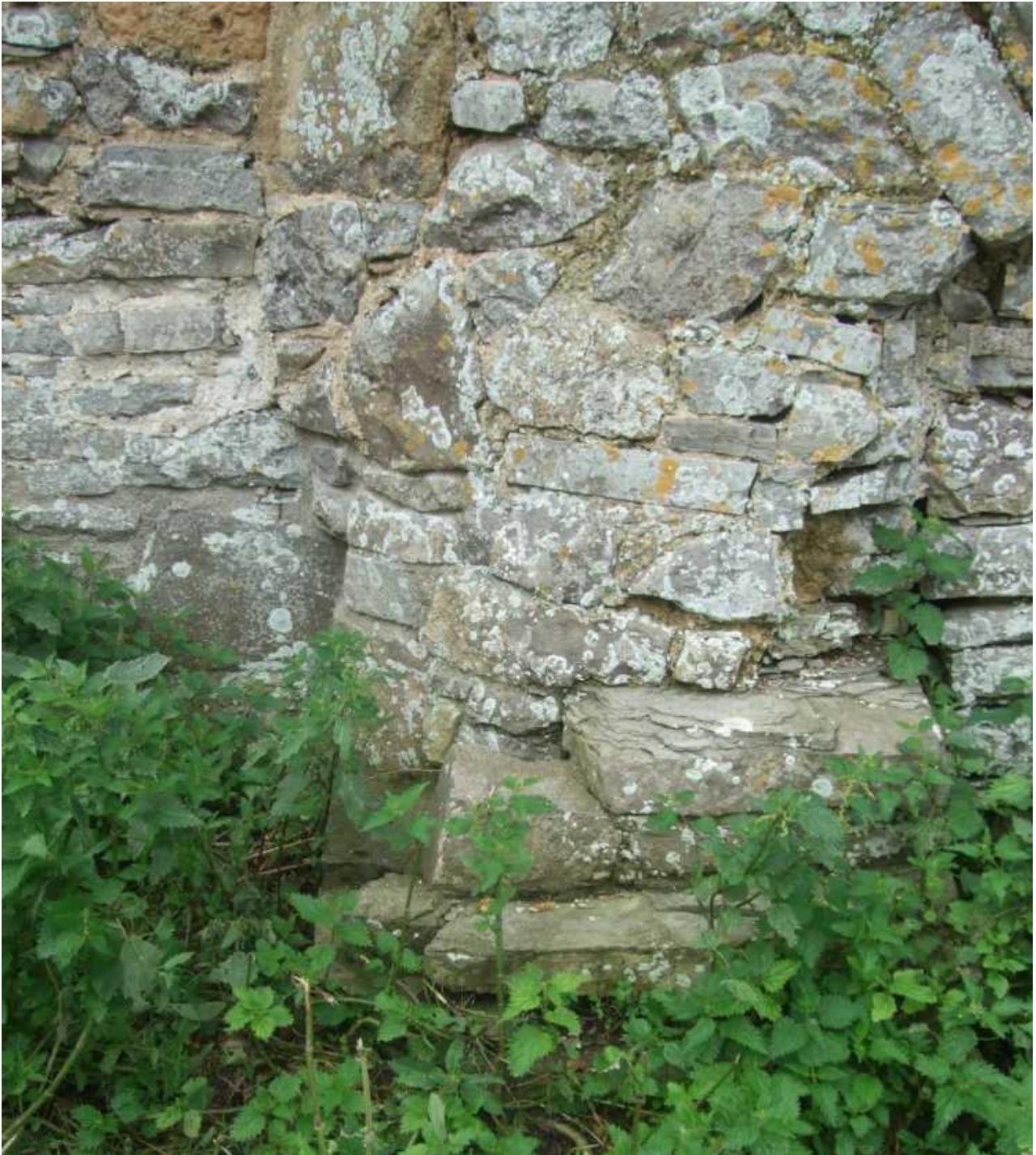
Fig 48: Junction of curved terminal to 'old' section of wall 7, and infill wall between it and wall 6
