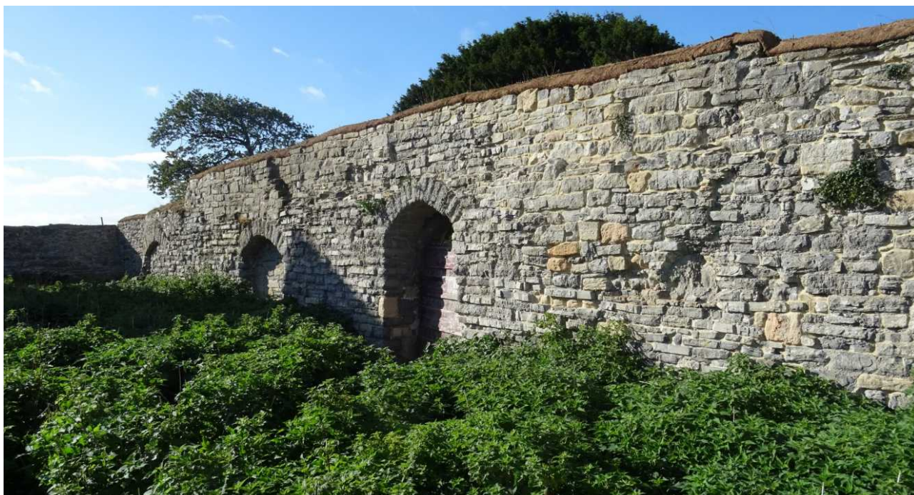
Fig 49: The upper stage of wall 7, clearly later, is thinner than the lower
