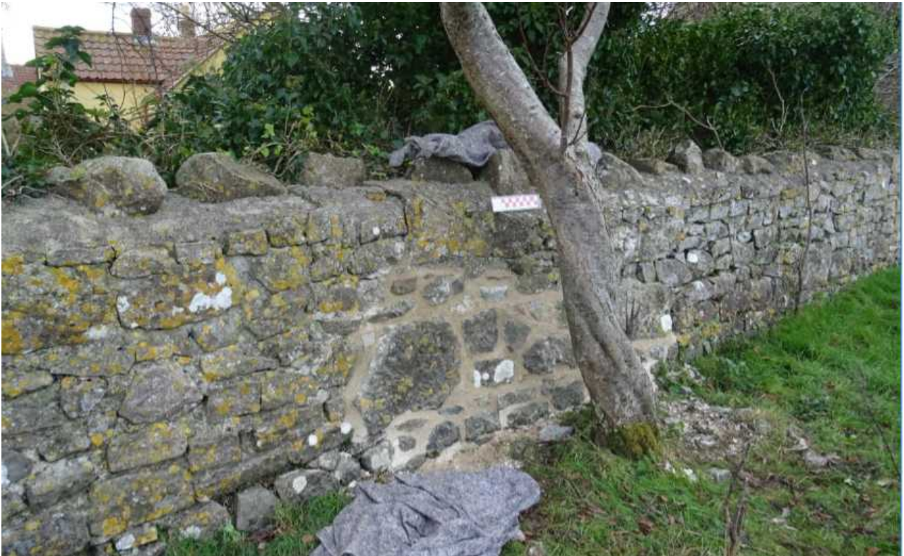
Fig 13: Wall 2 defect as repaired
