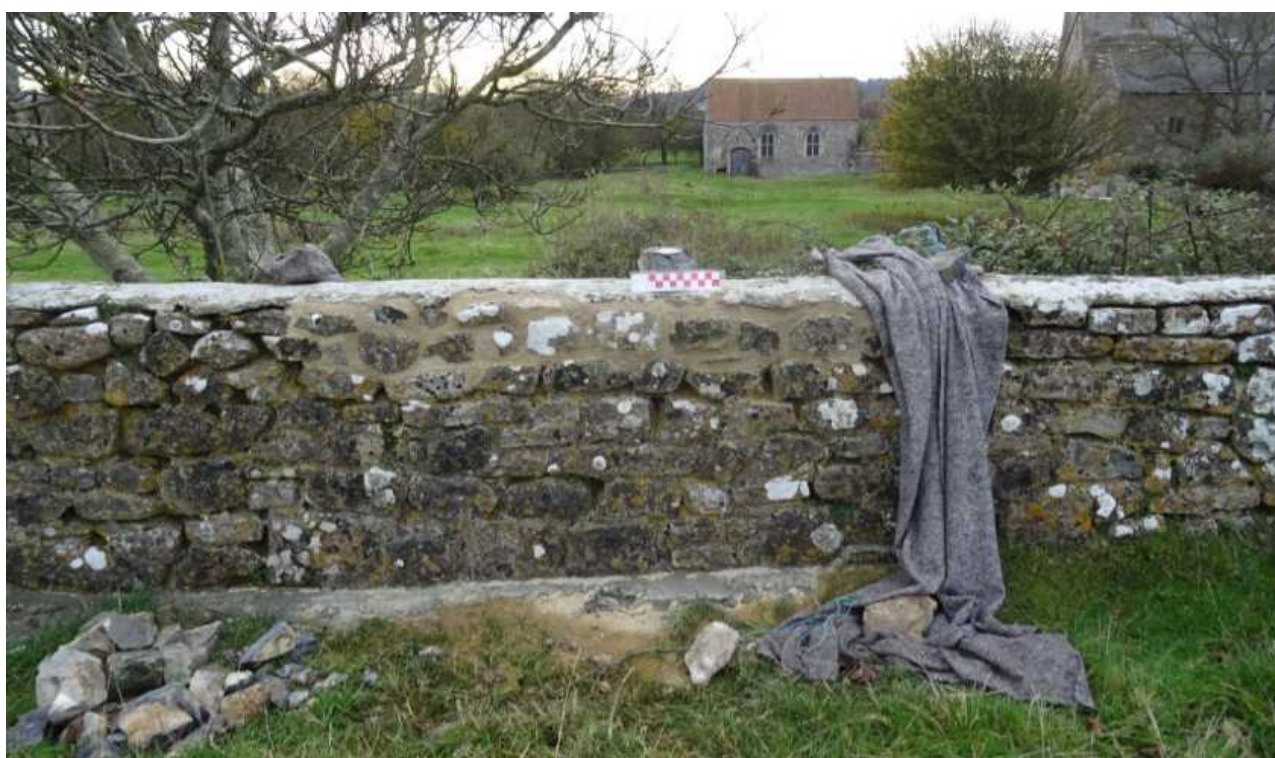
Fig 18: Minor defect as repaired and repointed November 2021
