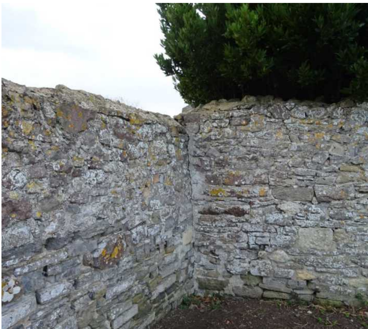
Fig 37: Butt joint of wall 7 (right) against north side of wall 6 (2021)
