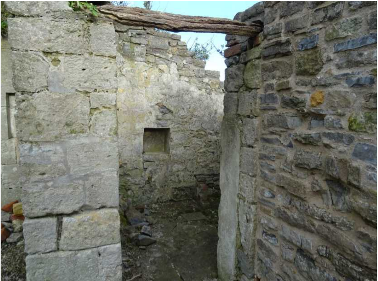
Fig 47: Thicker-walled structure at the northern end of wall 7, butted against the remaining chancel wall
