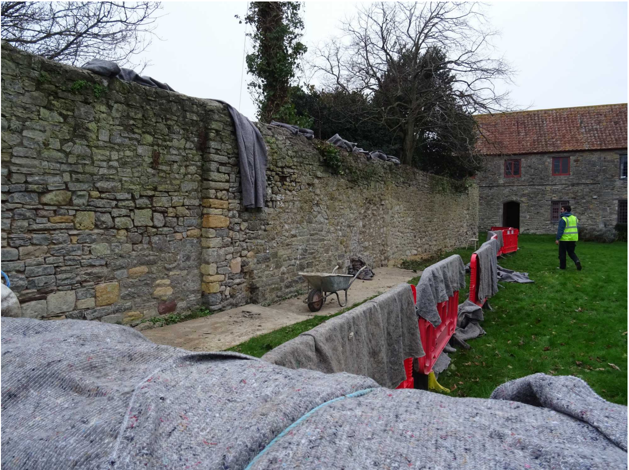
Wall 12/15 (west wall of garden) under repair and repointing, January 2022
