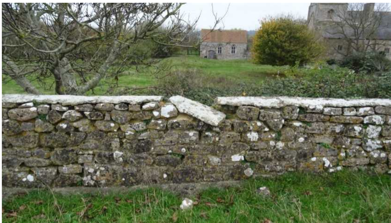
Fig 17: Minor defect in wall 3
