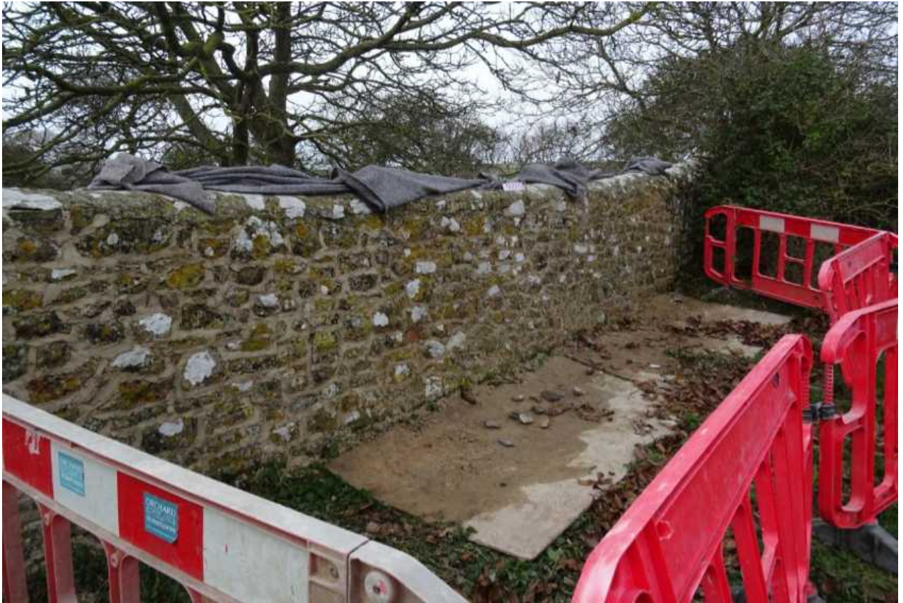
Fig 28: Subsequent repointing of exterior surface of wall 4
