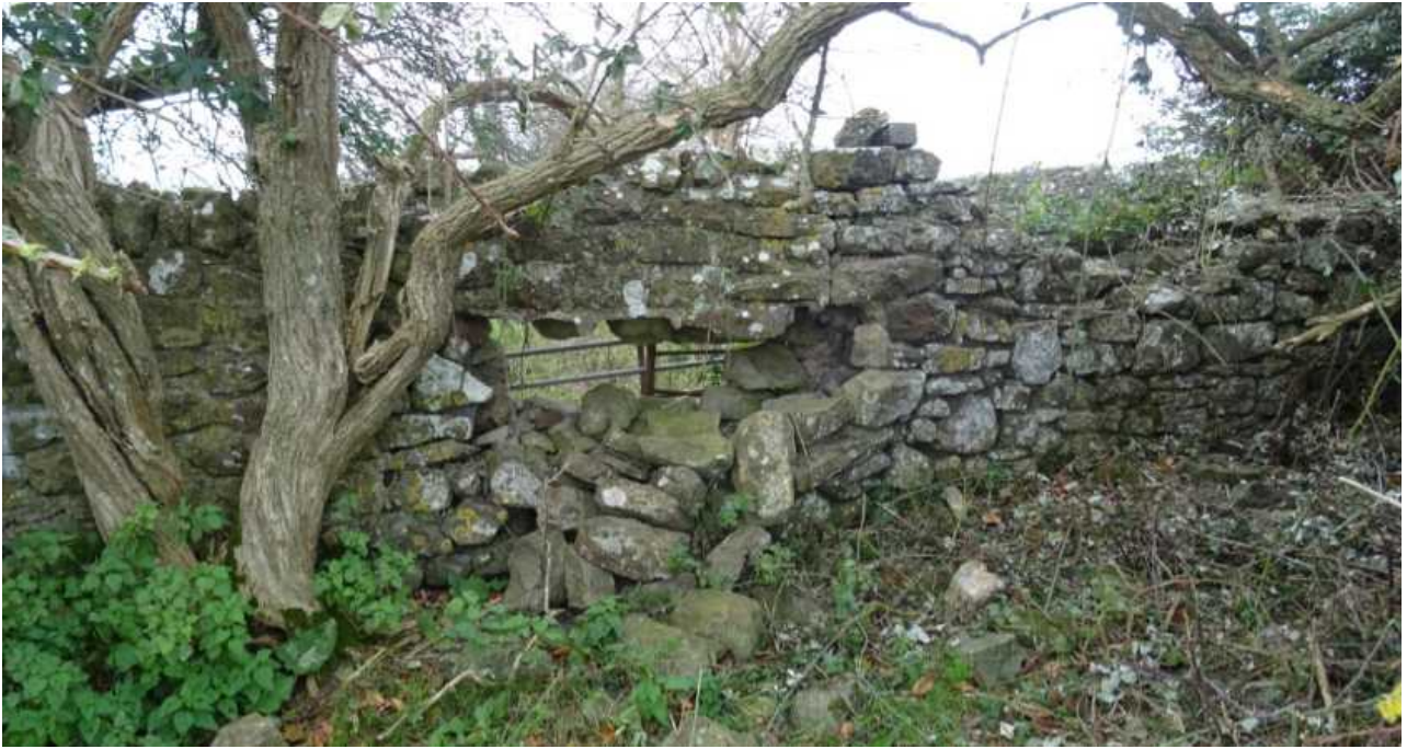
Fig 26: Collapse of wall in northern defect of Wall 4 (external view)
