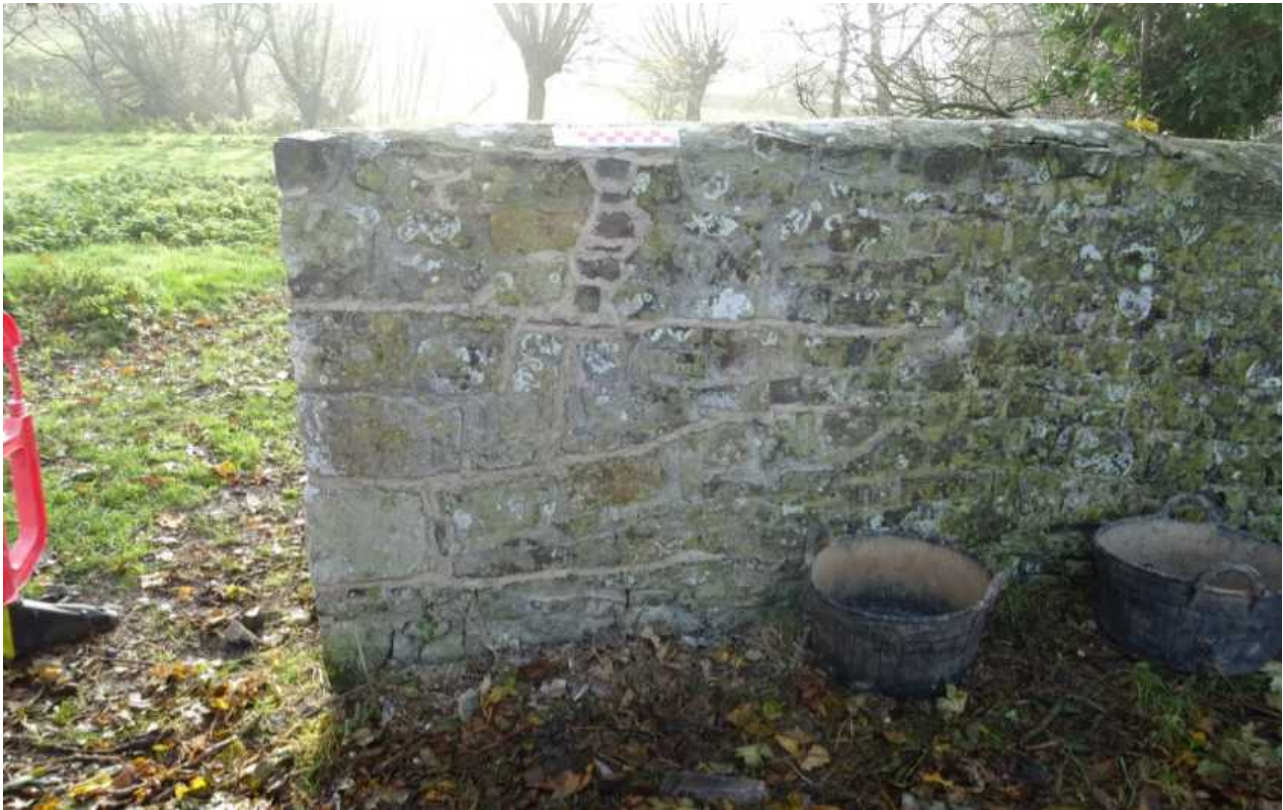
Fig 33: Wall 5: repointing of west jamb of field gate between orchard and outer fields
