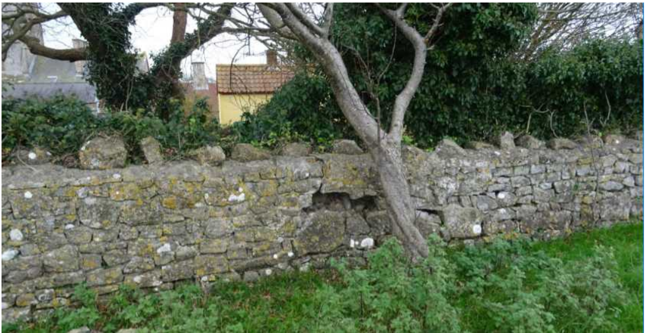
Fig 12: Defect in wall 2 (Woodspring Cottage is yellow building)
