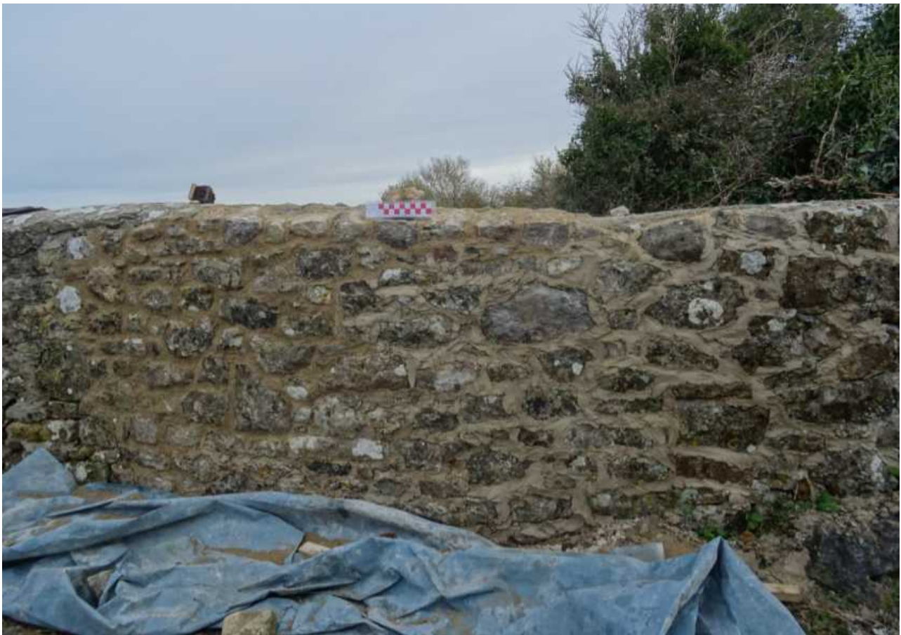
Fig 25: Wall 4 southern defect repaired and repointed
