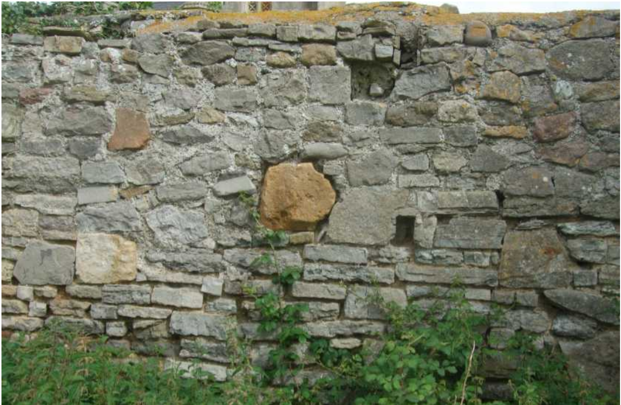
Fig 38: South side of wall 6, showing re-used freestone block and a socket (possibly two) for insertion of 20th century wooden structural members (2012)
