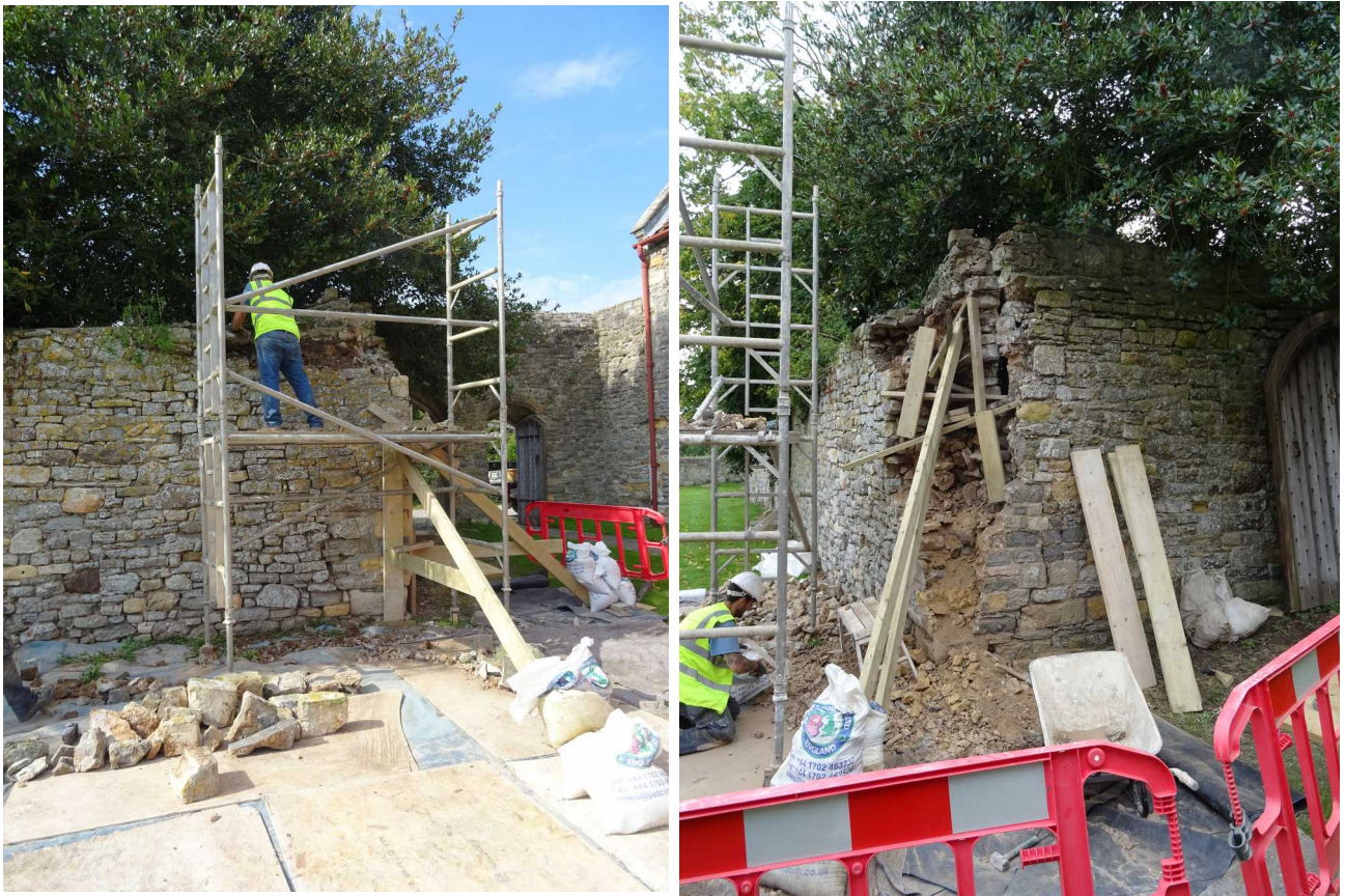
Fig 10: Increasingly complex propping as demolition proceeds
