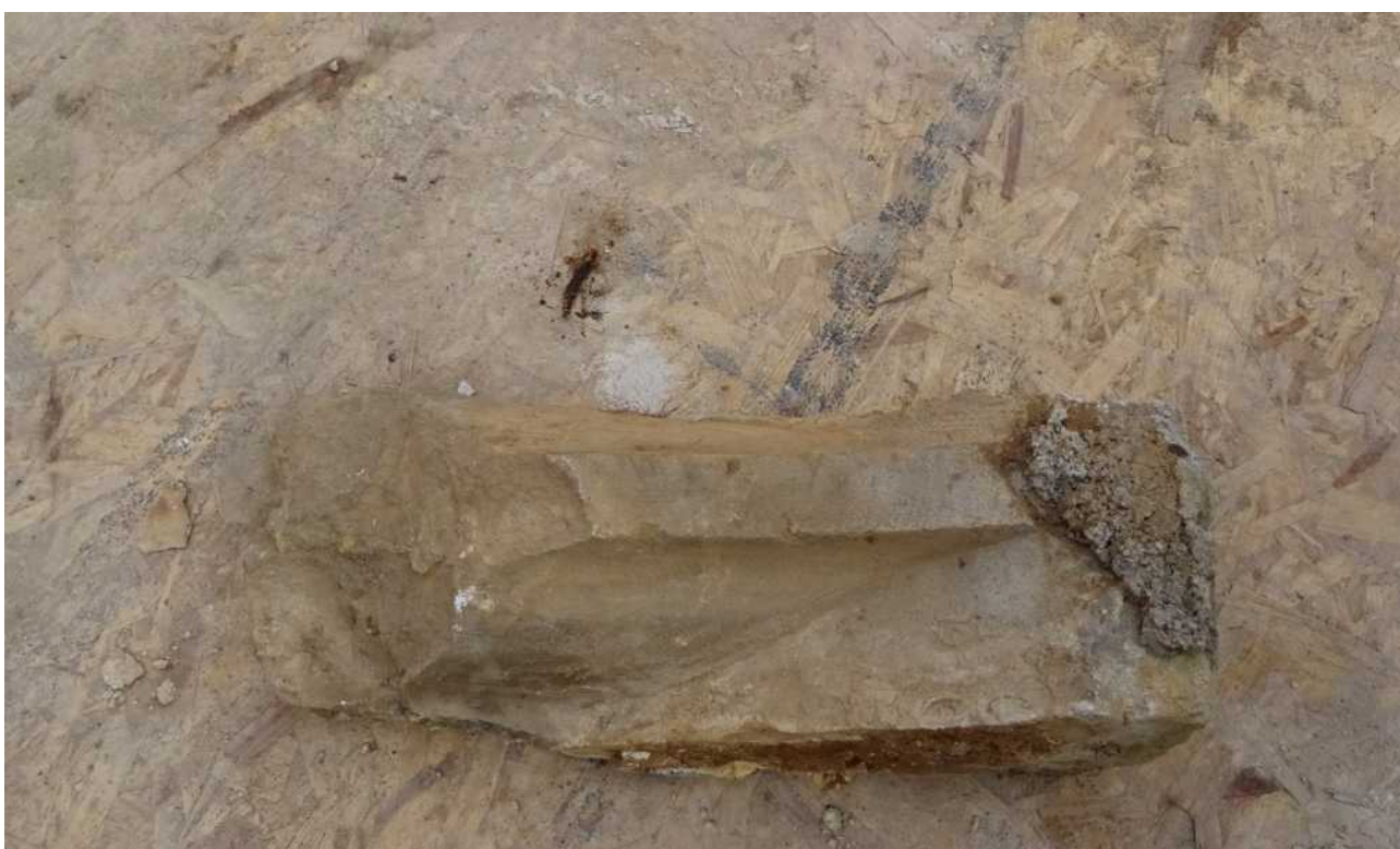
Fig 11: Section of ovolo-moulded widow column, with sloping sill (approximately 45cm long)
