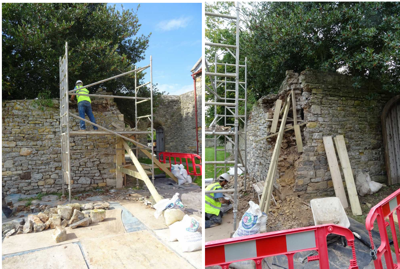
Fig 10: Increasingly complex propping as demolition proceeds
