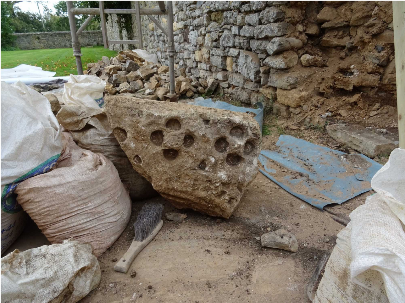
Fig 13: Upper right corner of Tudor fireplace, with quatrefoil settings, corner vegetative spandrel and apparent 4-centred mouldings. Re-used as lowest quoin in the corner of the wall, where it can be clearly seen in Figs 8 and 9
