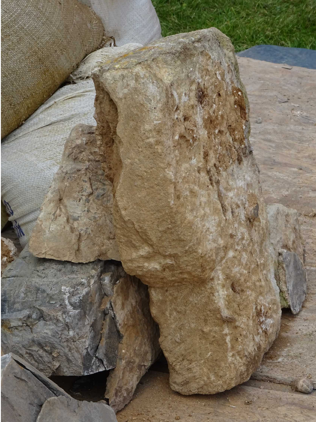
Fig 12: Freestone block with rebate: possibly a column base or plain corbel: re-used in wall as quoin. Length 45cm.
