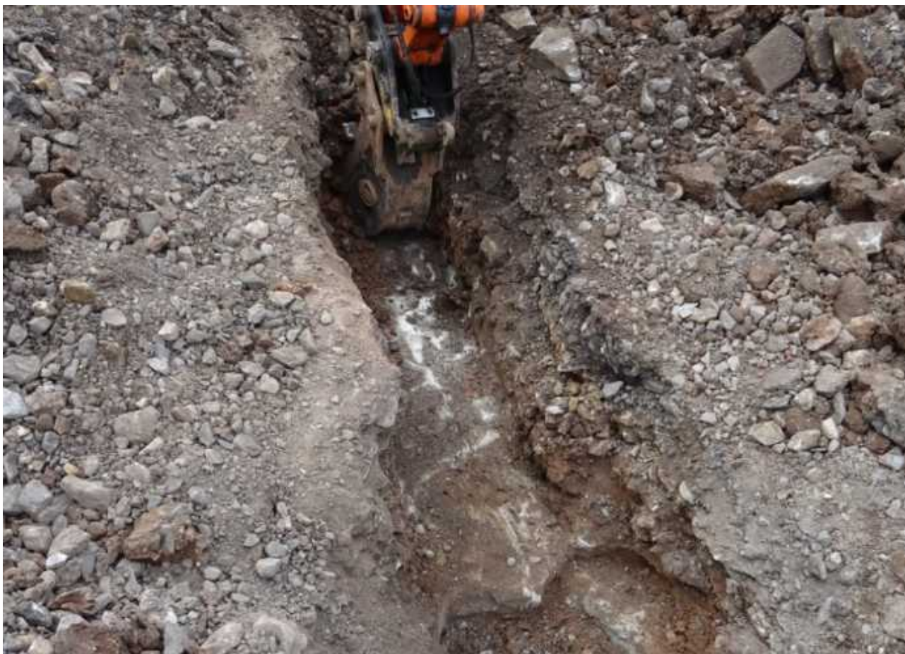
Fig 8: Pennant Sandstone slab in trench before breaking up (12 April 2018)
