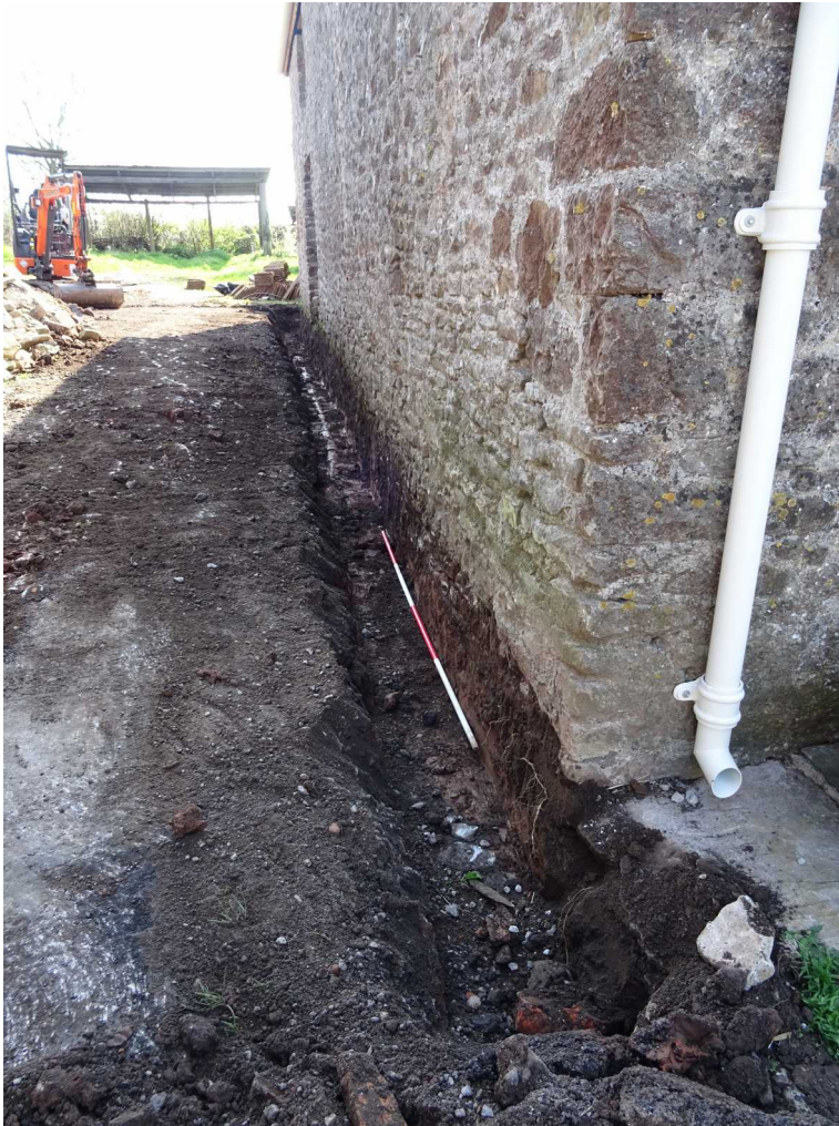
Fig 6: Trench beside north-east range of buildings, 12 April 2018
