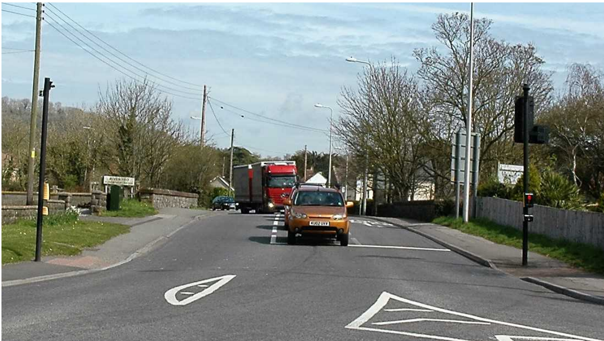
Fig 22: The Bridge today
