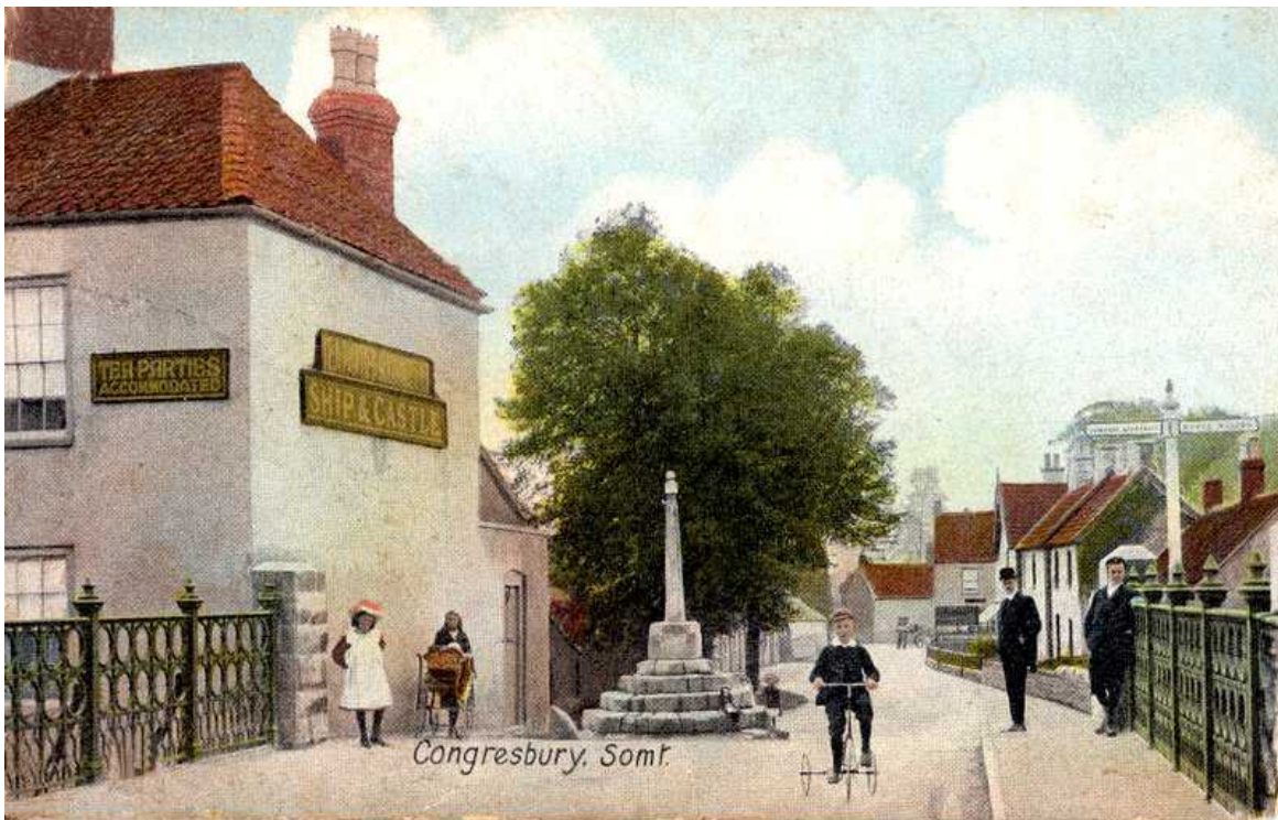
Fig 4: The bridge following the repairs & alterations. Courtesy of Congresbury History Group
