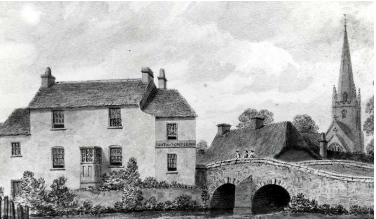
Fig 2: Drawing by Buckler 1828 (Somerset Archaeological and Natural History Collections) The 1710 stone bridge by this time had been widened, in 1817 by Edward Lukins.
