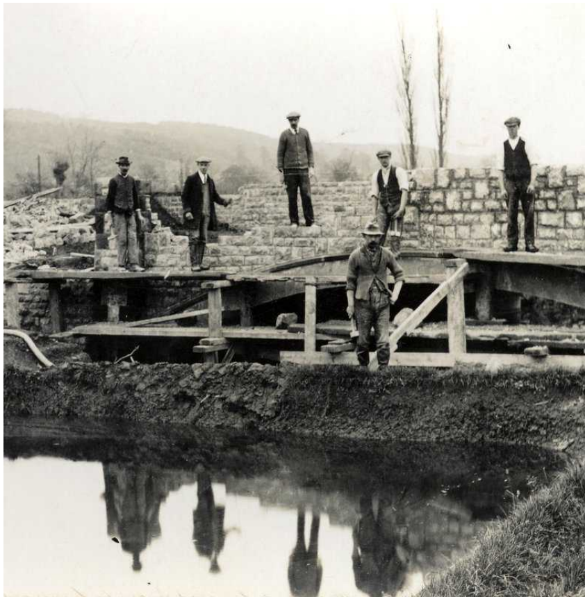
Fig 10: 1924 construction looking towards Cadbury Hill. Courtesy of Congresbury History Group
