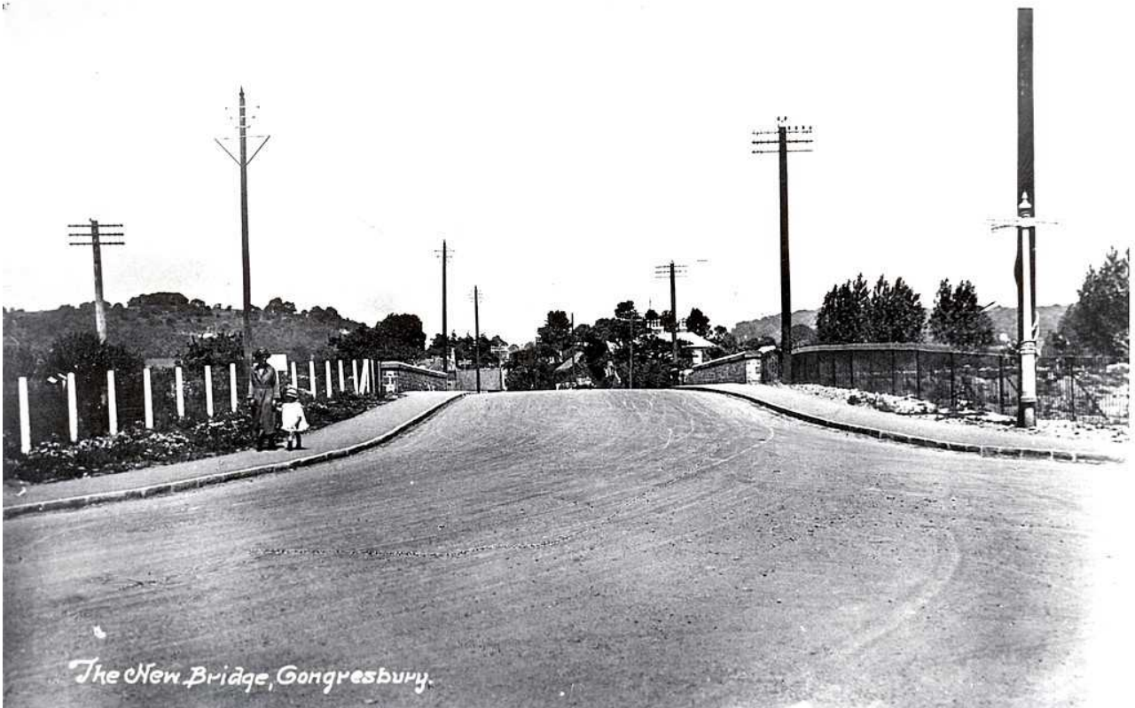
Fig 15: New bridge c1924 looking north
