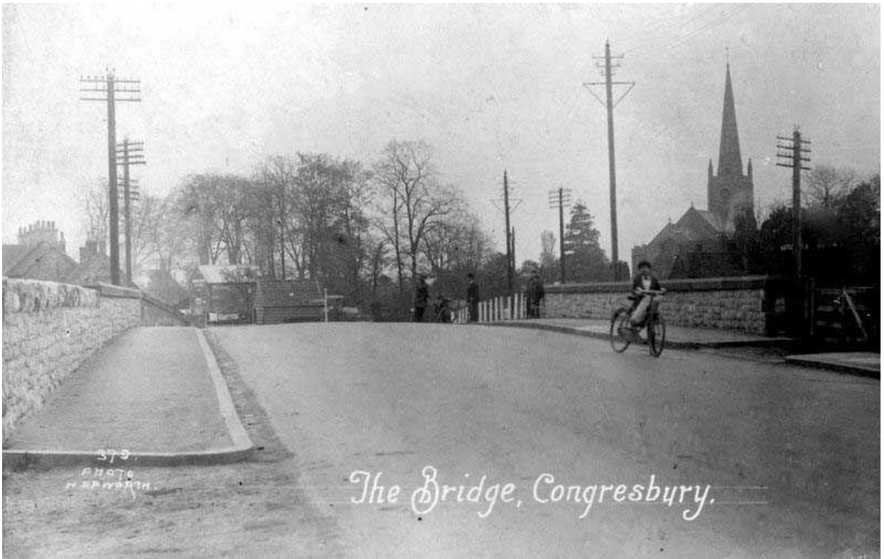
Fig 14: Alf Sampson photo of new bridge looking south. According to John Walter the first person to drive over the bridge was "Lucky" Stevens who lived by the Elms
