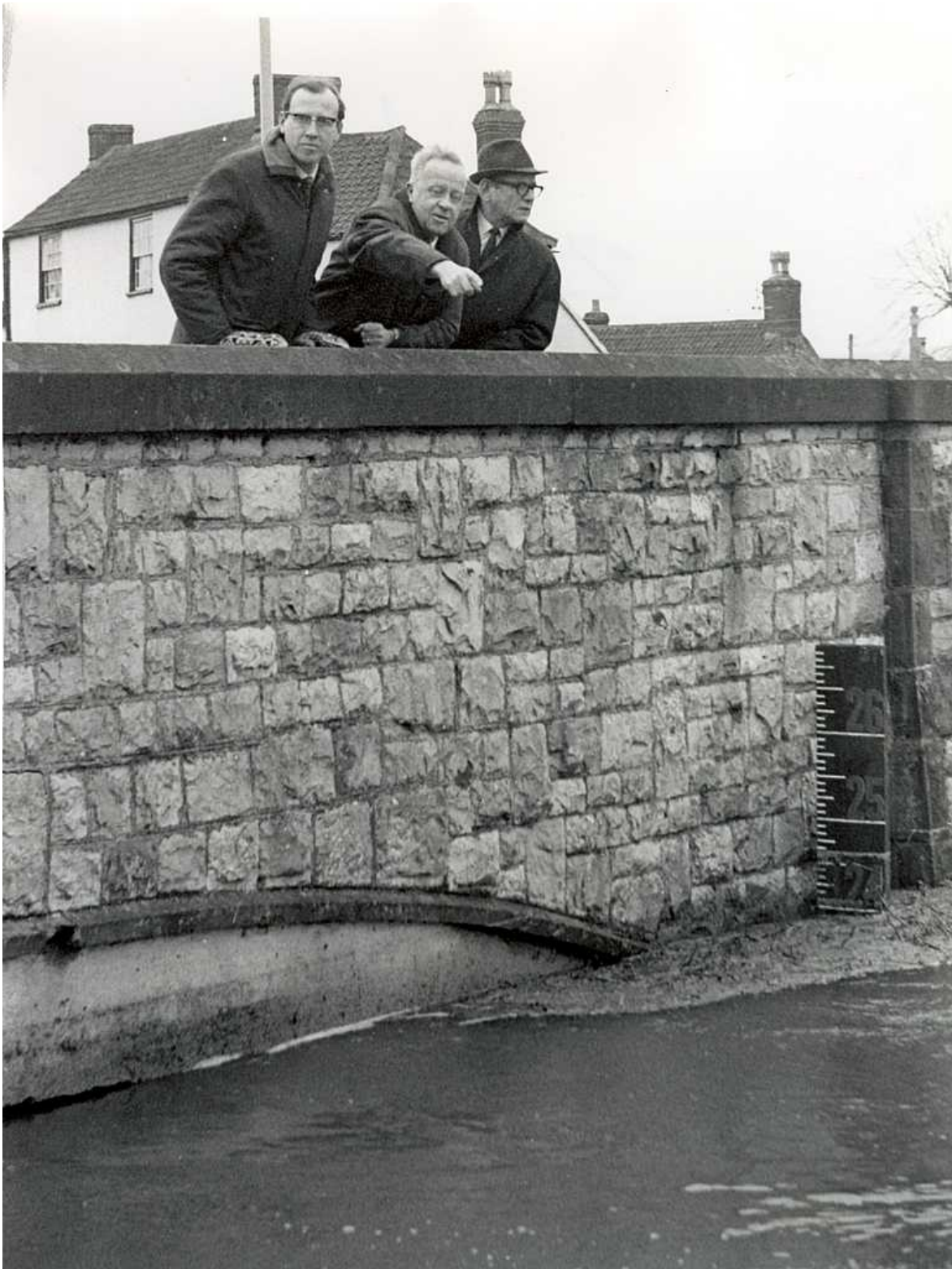
Fig 18: July 1968: Derrick Cox left & J Walter centre
