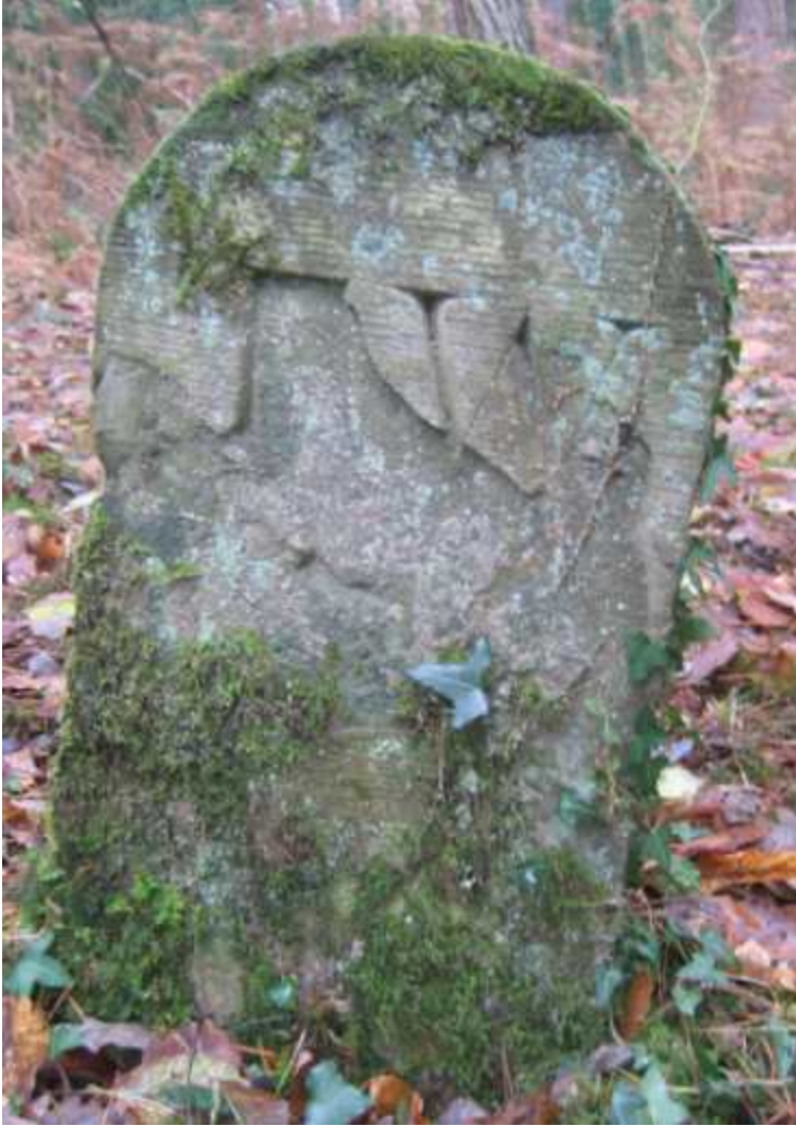
Fig 8: Stone 9 at Woolmers showing typical shaling damage
