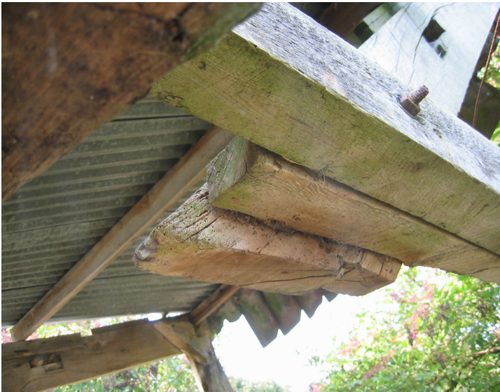
Fig 12: Sawn-off foot of re-used truss
