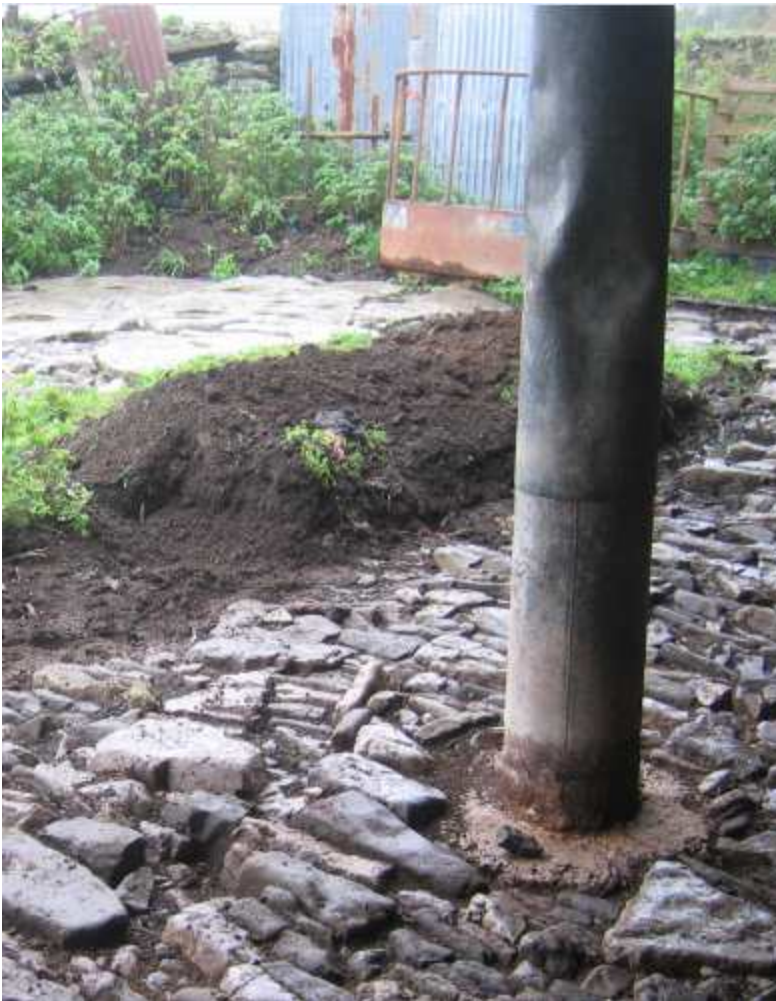
Fig 14: Cylinder holding up the roof structure of the eastern building
