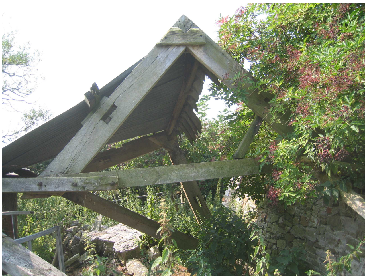
Fig 11: Collapsing roof structure of western building, August 2005. Note the re-used elements
