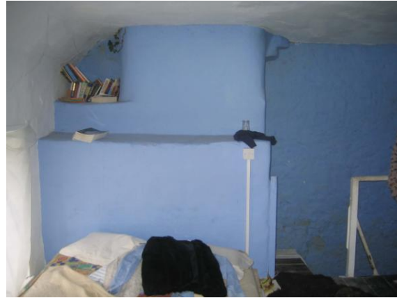
Fig 7: Stack on first floor - top of stair to right
