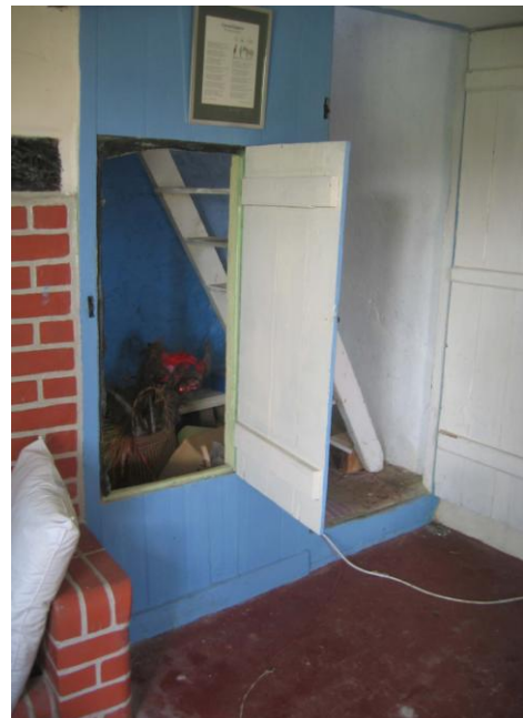
Fig 5: Open stair in cupboard
