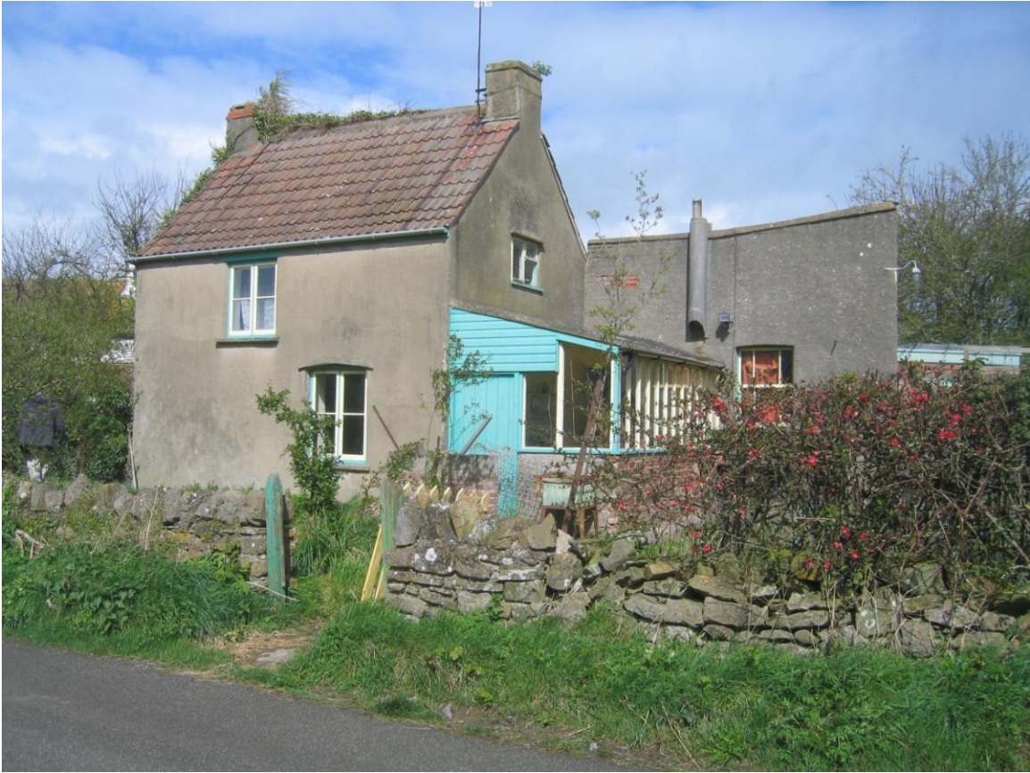
Fig 3: Cottage from the road, extensions to right of picture. Note false stack to right gable.
